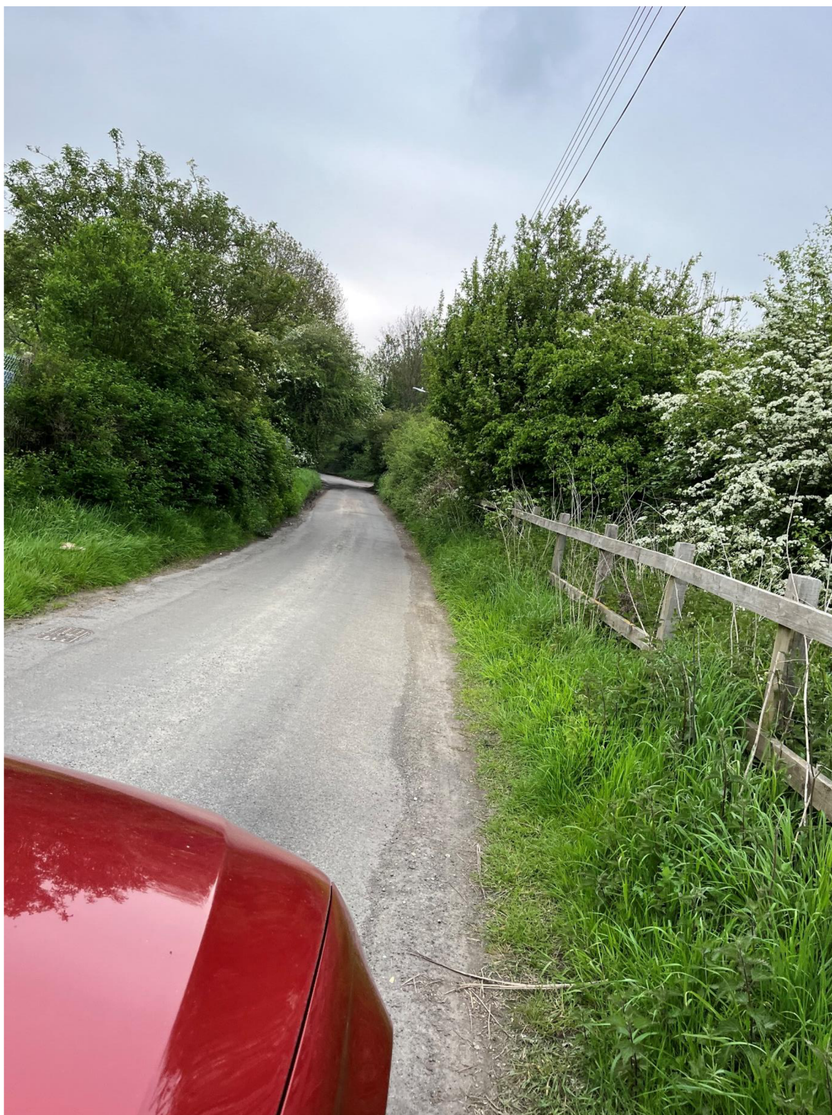
Along Downs Road Towards Instead Rise
