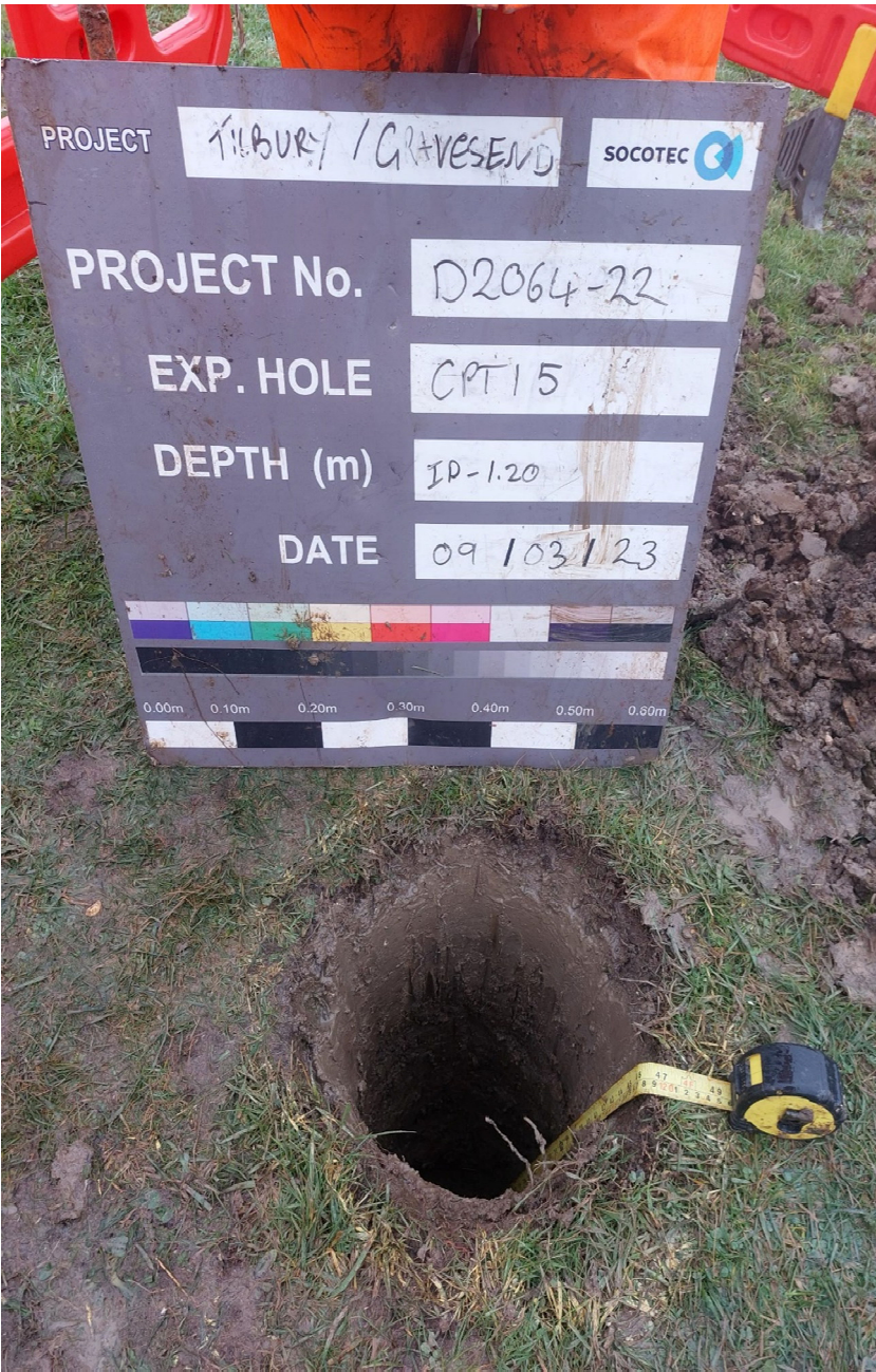
CPT15 – Inspection pit – 0.00m to 1.20m
