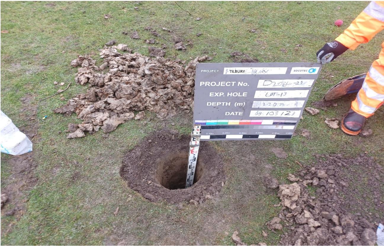
CPT13 – Inspection pit – 0.00m to 1.20m
