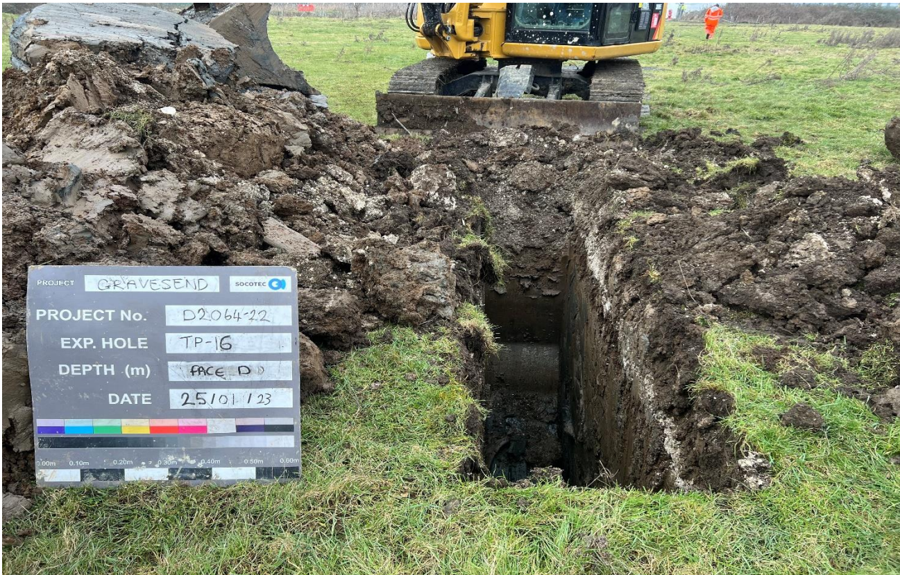
TP-16 Face D & Spoil
