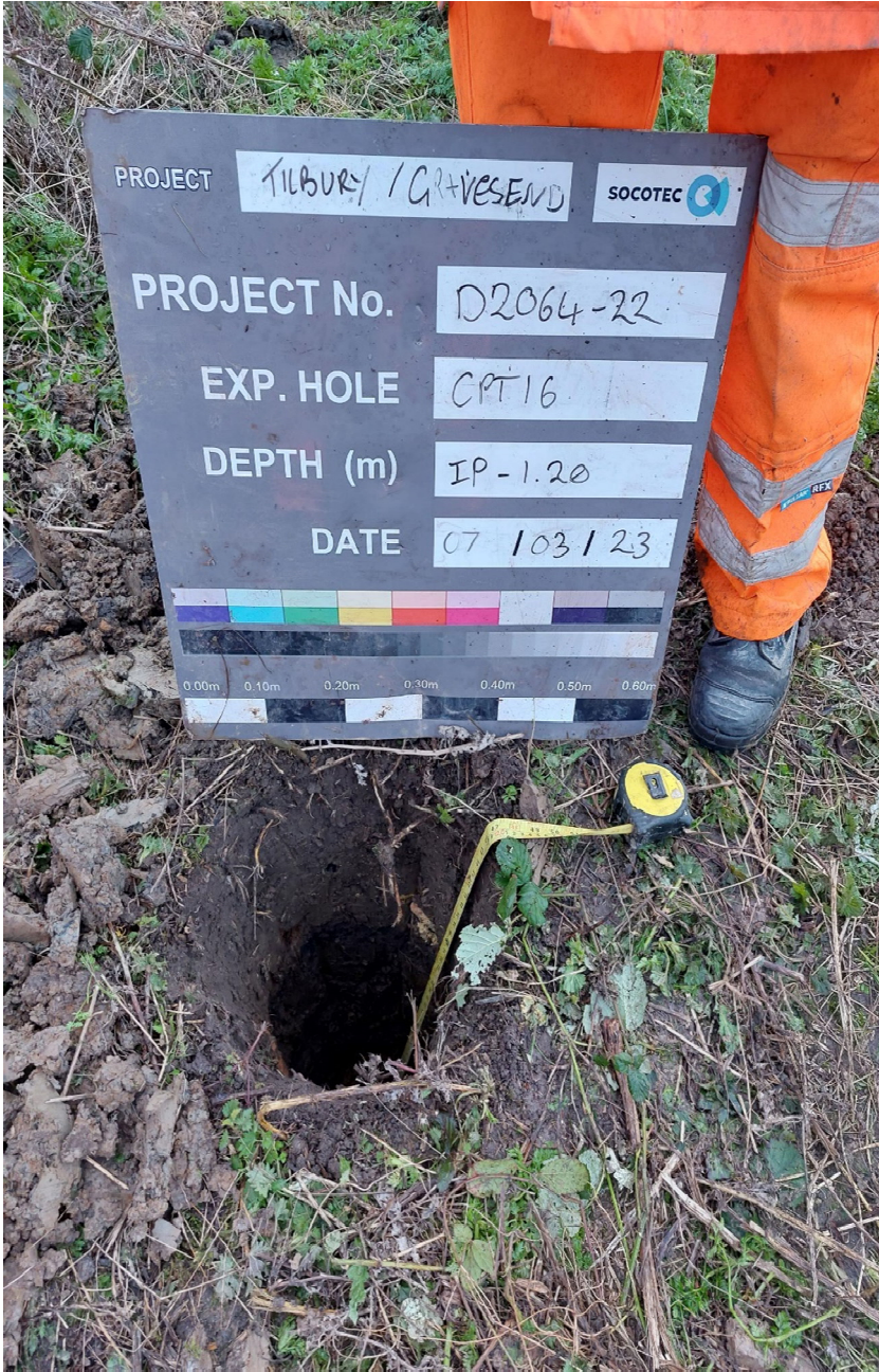
CPT16 – Inspection pit
