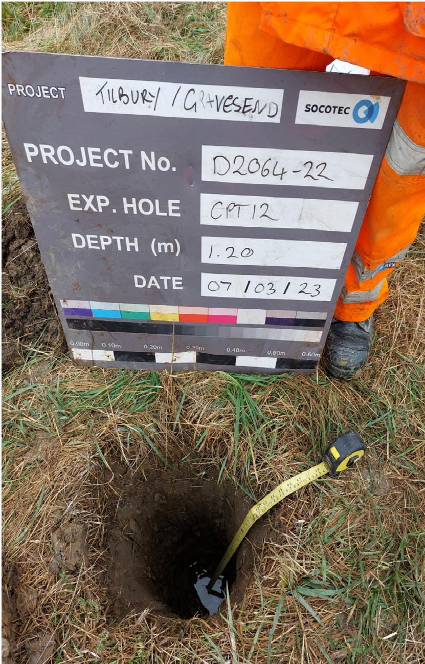
CPT12 – Inspection pit – 0.00m to 1.20m
