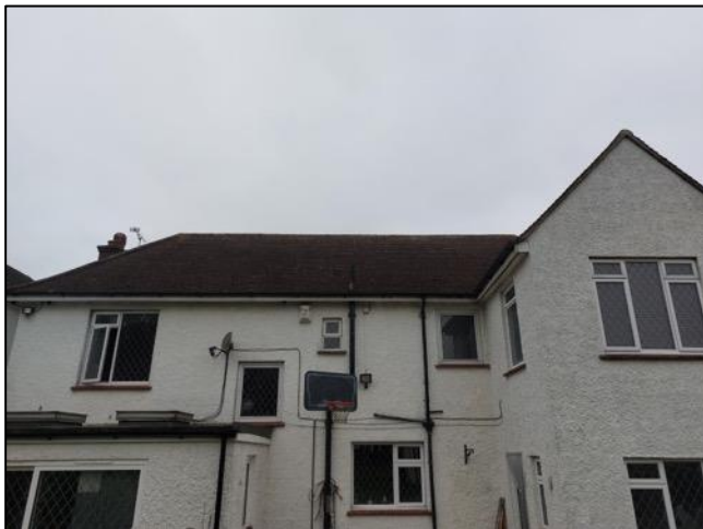
Photograph 1. Overview of the rear elevation.
