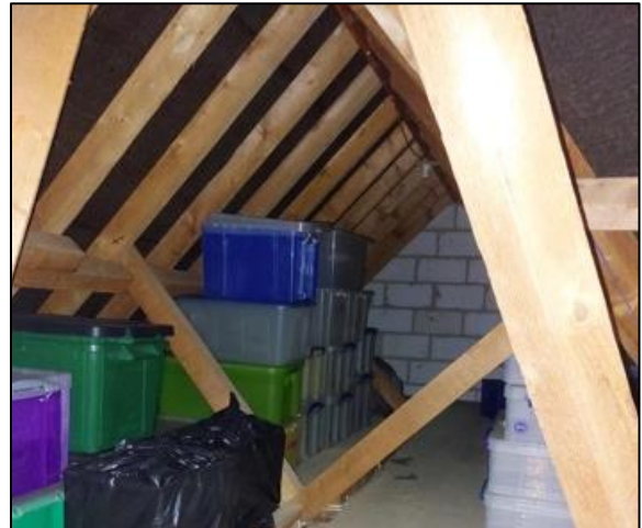
Photograph 8. Internal loft void.
