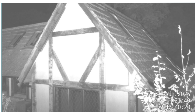
Photograph 8. NVA view of survey position S5
