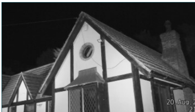
Photograph 6. NVA view of survey position S3
