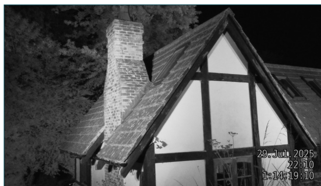
Photograph 9. NVA view of survey position S6
