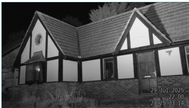
Photograph 4. NVA view of survey position S1
