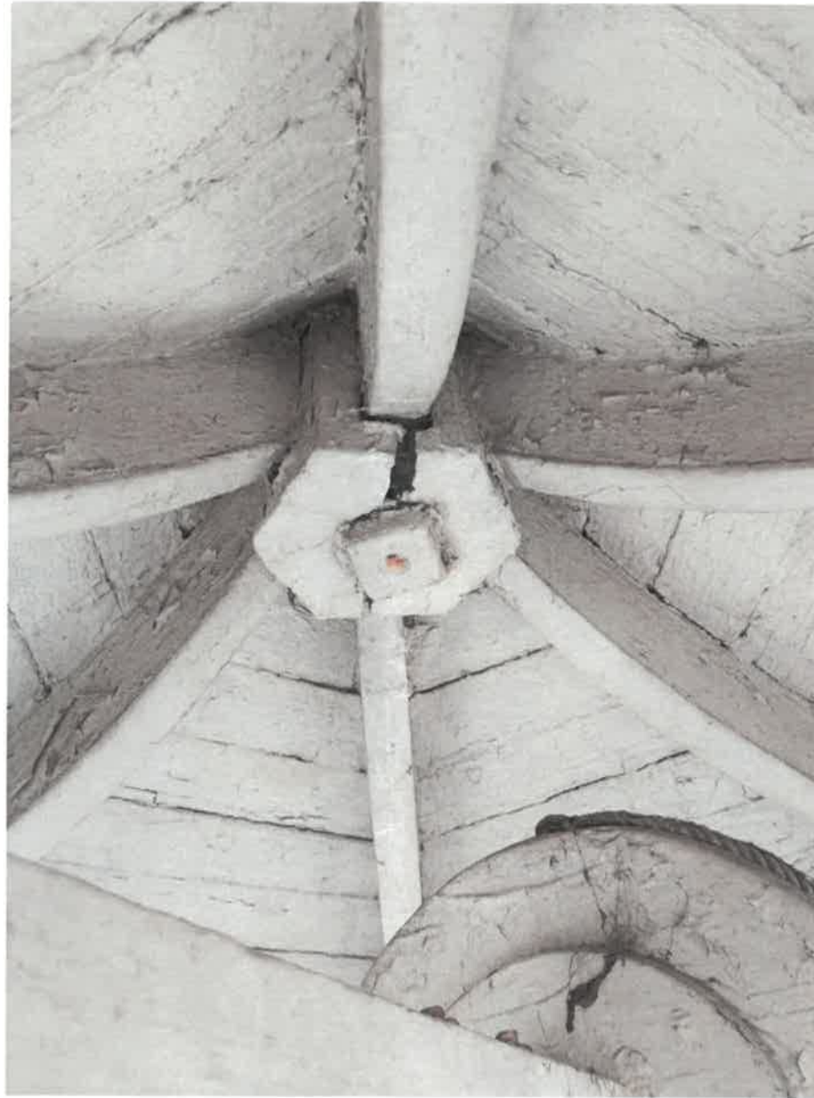
3) Underside of cupola HCPX01.
