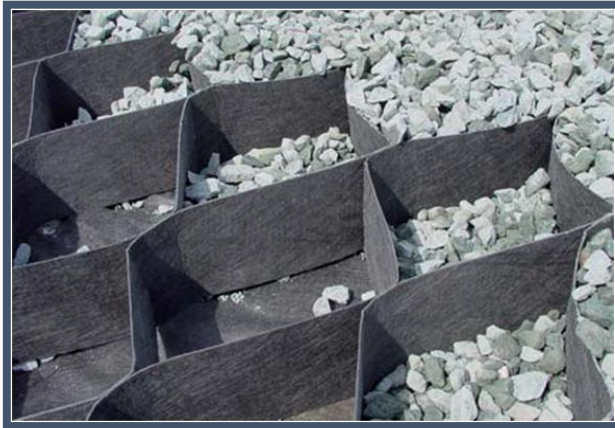
Figure 10 Examples of Cellweb filling with angular stone
