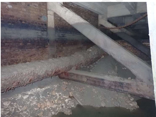
Photo 11 – View of internal structure of wall 1
