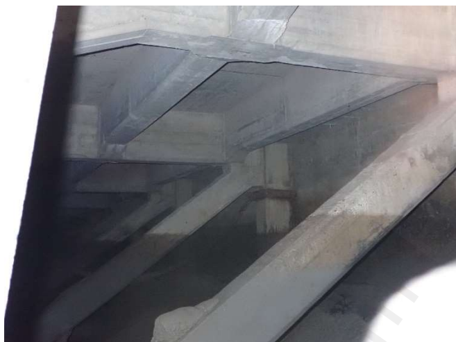
Photo 15 - View of internal structure showing the concrete beams and Masonry wall through wall 1
