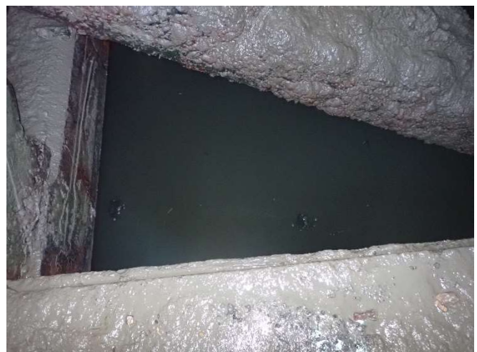
Photo 12 - View of internal structure of wall 1
