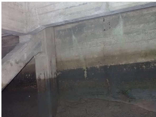
Photo 13 - View of internal structure of wall 1
