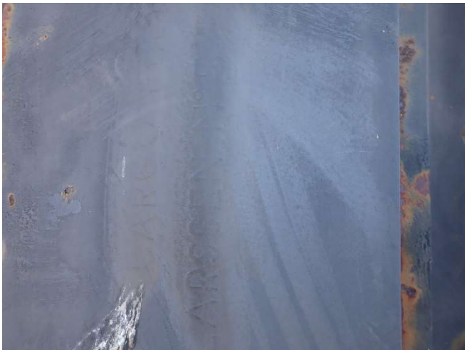
Photo 9 – Typical view of Larssen N°5 pile
