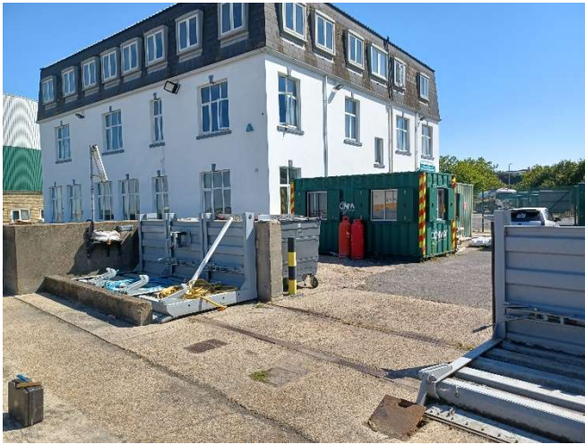
Photo 7 – General photo of flood gate
