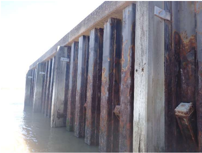
Photo 47 - General view of wall 3 fenders
