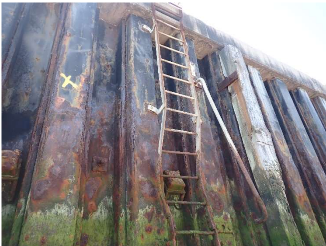
Photo 37 – General view of ladder 2 on wall 2
