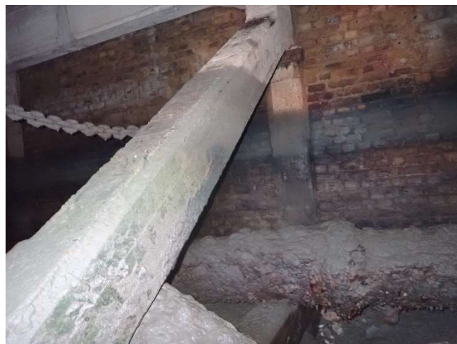
Photo 14 - View of internal structure of the masonry wall through wall 1
