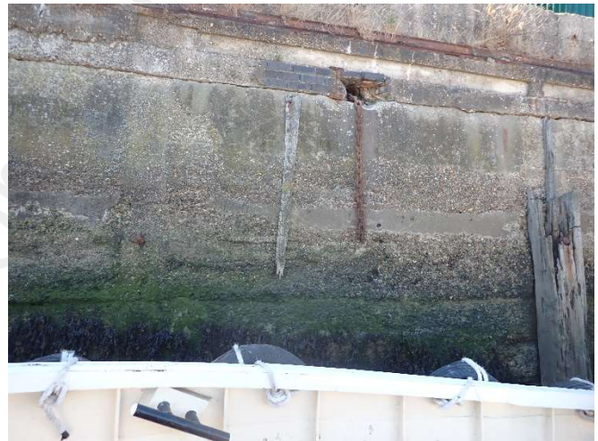
Photo 32 – View of wall 1 brickwork
