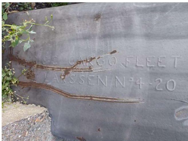
Photo 17 – Typical view of Larssen N°4-20 sheet
