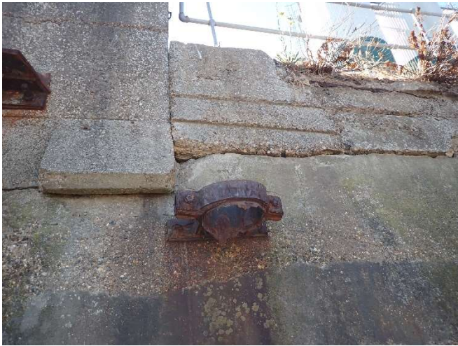
Photo 29 – View of remains of steel pipe on wall 1
