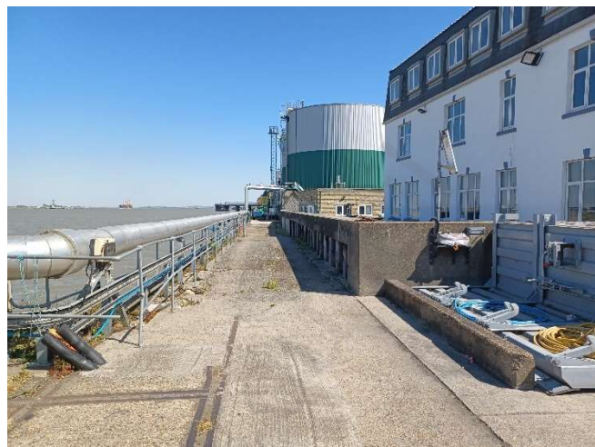
Photo 18 – View of downriver flood defence wall from the floodgate
