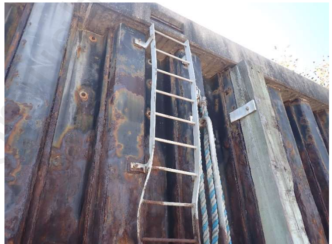
Photo 38 – General view of ladder 3 on wall 2
