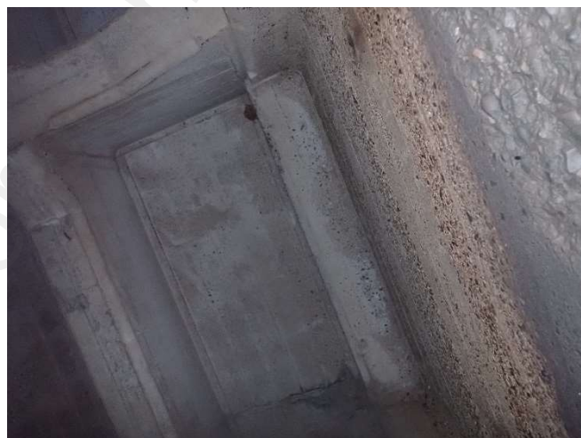
Photo 16 - View of internal structure of wall 1
