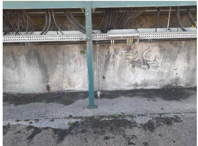
Photo 52 - View of calcite deposit on wall 5
