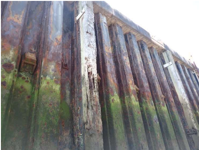
Photo 41 – Typical view of wall 2 fender
