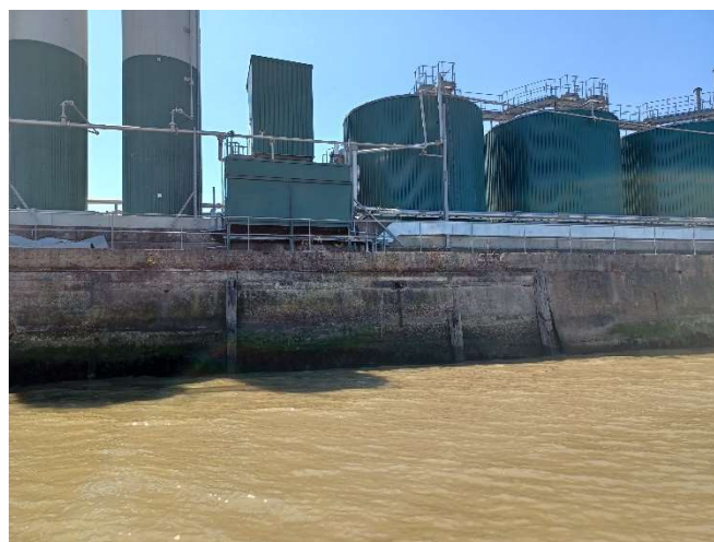
Photo 22 – View of wall 1 fenders
