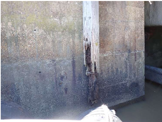
Photo 31 – View of wall 1 timber fender
