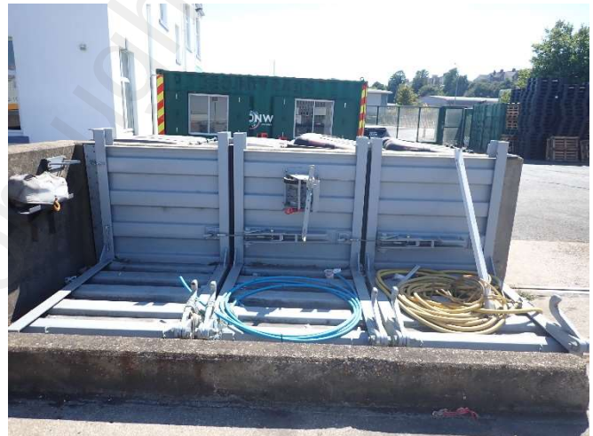
Photo 10 – General view of downriver flood gate
