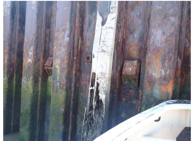
Photo 42 – Typical view of wall 2 fender
