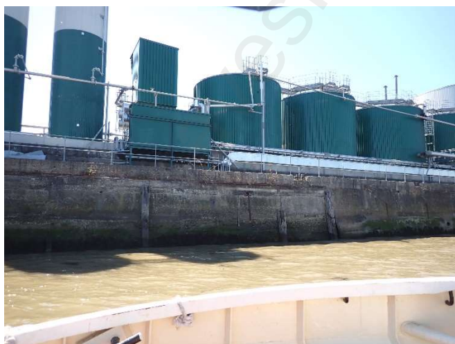
Photo 21 – View of wall 1 fenders
