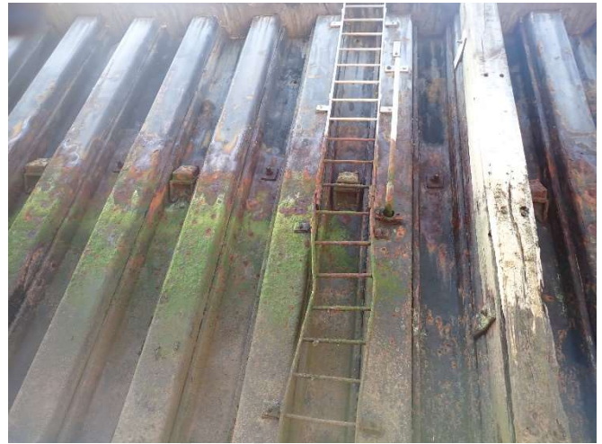
Photo 36 – General view of ladder 1 on wall 2
