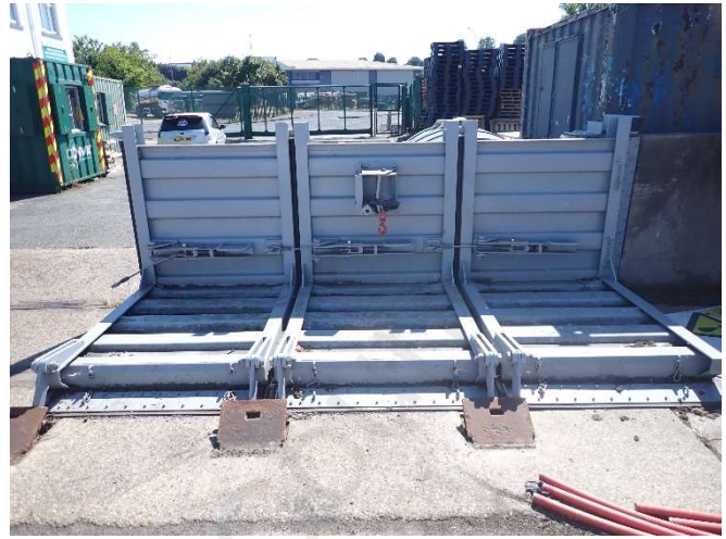
Photo 8 – General view of upriver flood gate
