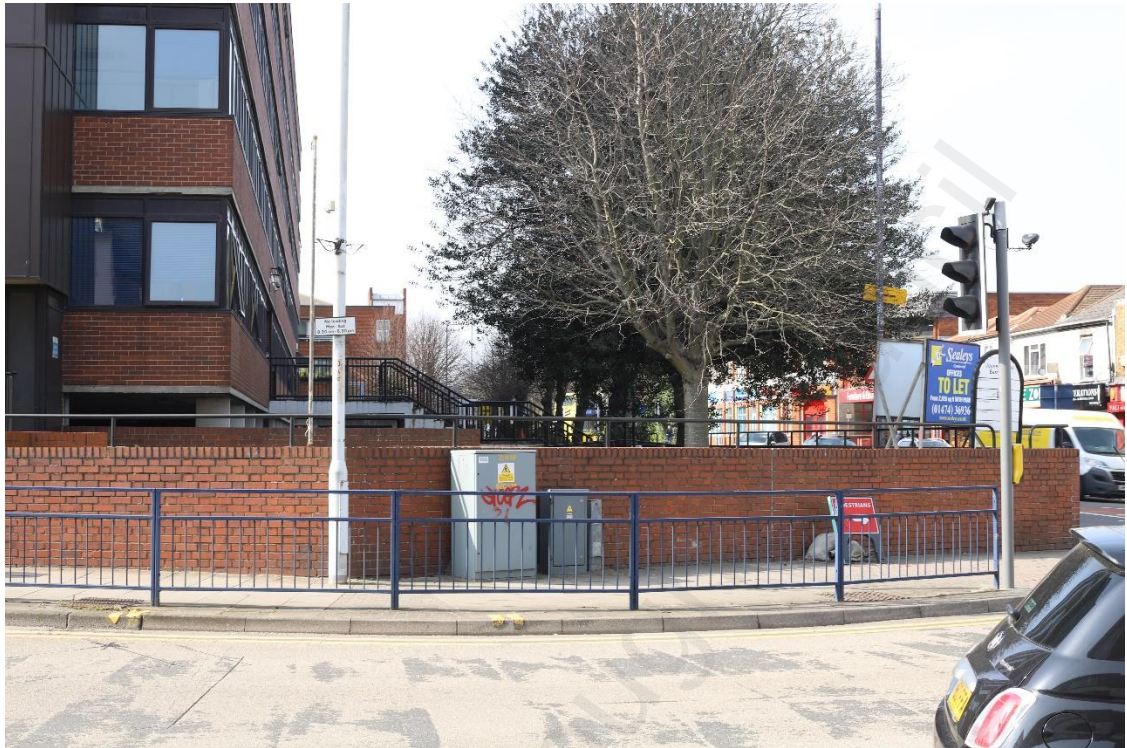
Plate 3 Joynes House, perimeter wall along the eastern edge and trees along the A226 / New Road.
