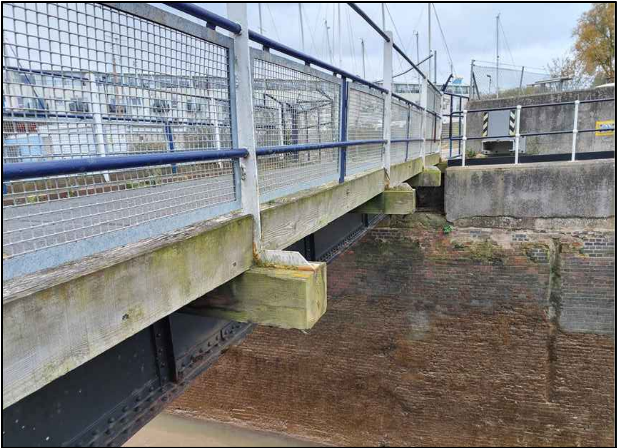
PHOTO 1 - ELEVATION TO SIDE OF EXISTING BRIDGE
