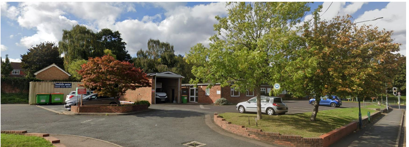
View of library site to north
