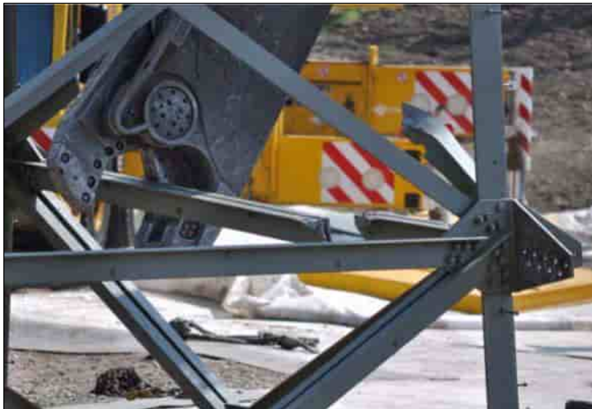
Plate 3-16: Hydraulic Shearer Mounted on an Excavator Boom
