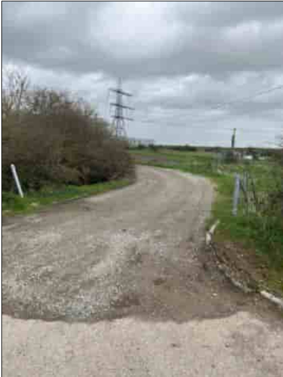
Plate 3-22: Access Road to the Gravesend site from the Thames and Medway Canal Road
