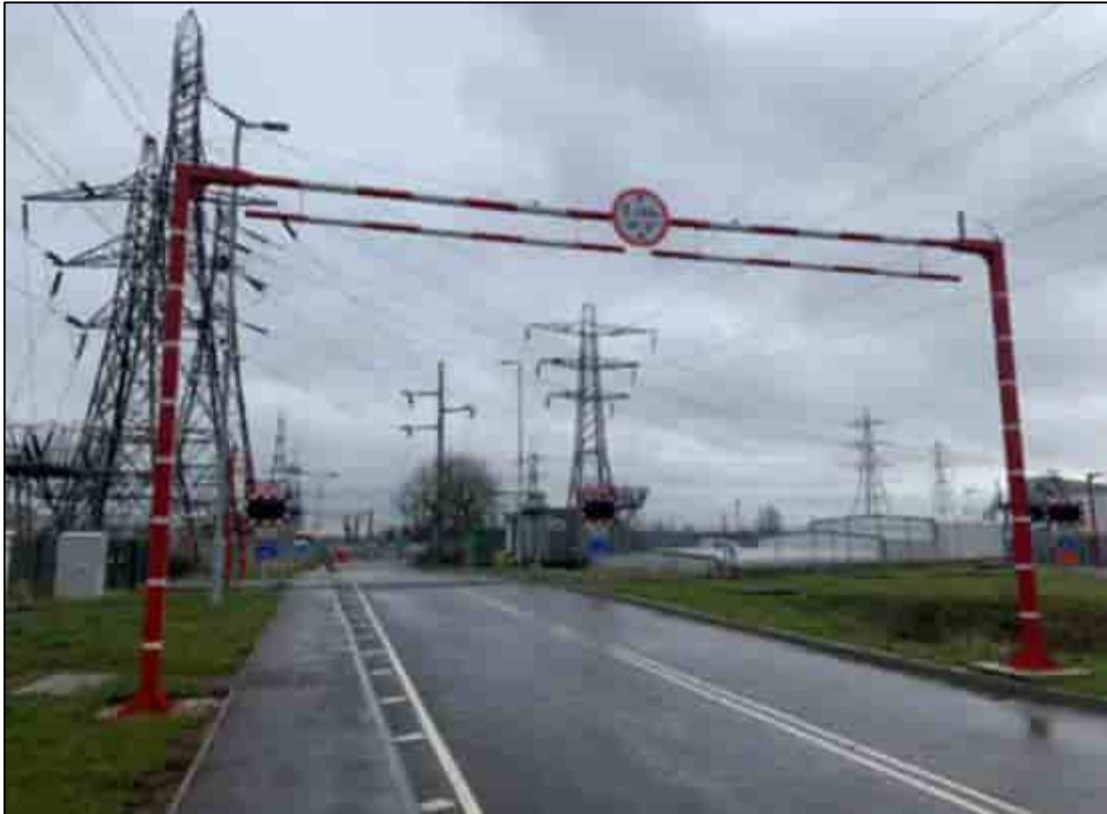
Plate 3-17: Rail Crossing Height Restriction at TQ 65959 76076
