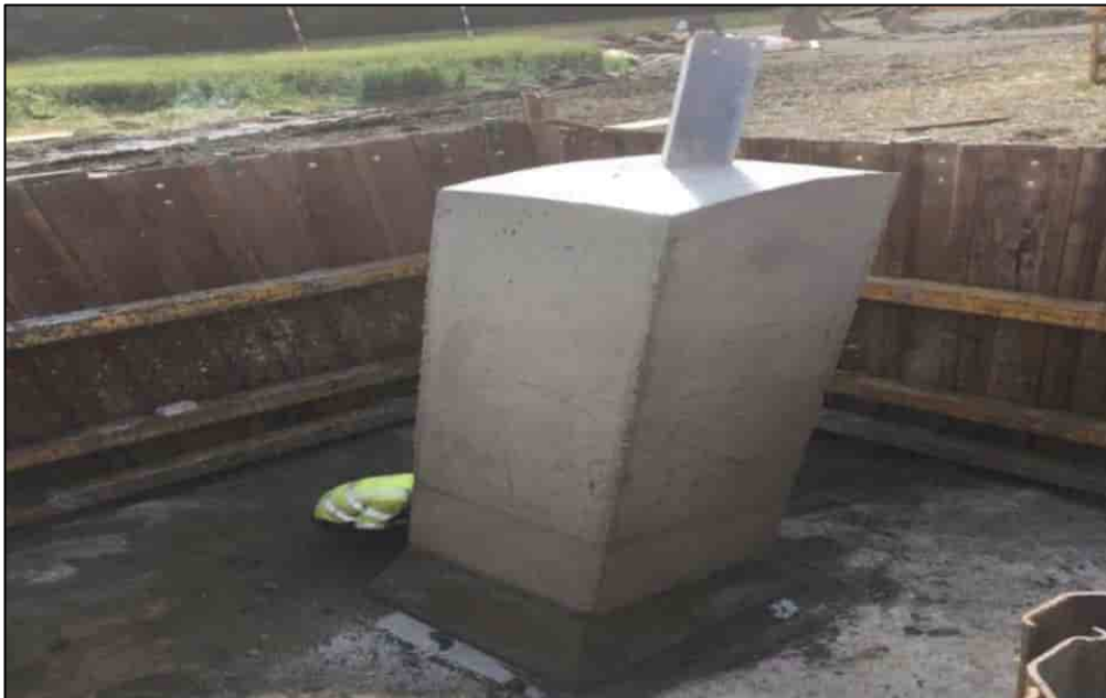
Plate 3-15: Typical Excavations for Upgrading of Pylon Footing Foundations
