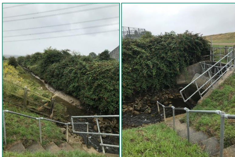
Plate 21-1: Photos 12G (left) and 12H (right) – GS2 and sluice gate taken during site visit
