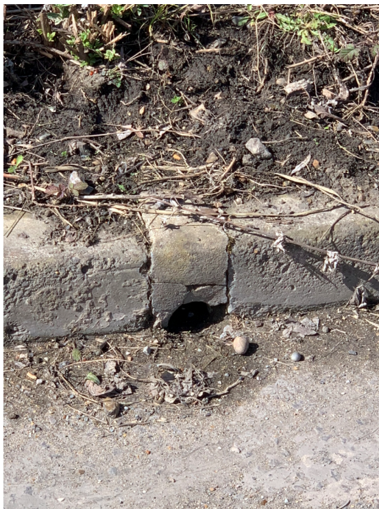
Figure 1: Tilbury existing road drainage.
