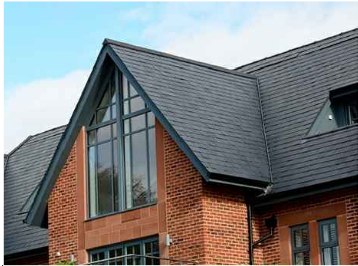
Natural slate roof
