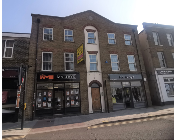
Fig 04 - Numbers 17 and 19 Stone Street, ground floor commercial space with vacant office space above over first and second floors.
