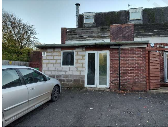
Fig 2. Photo to the rear
