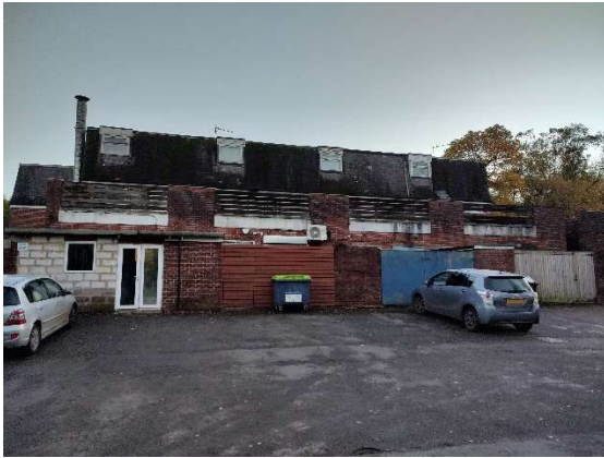
Fig 1. Photo to the rear
