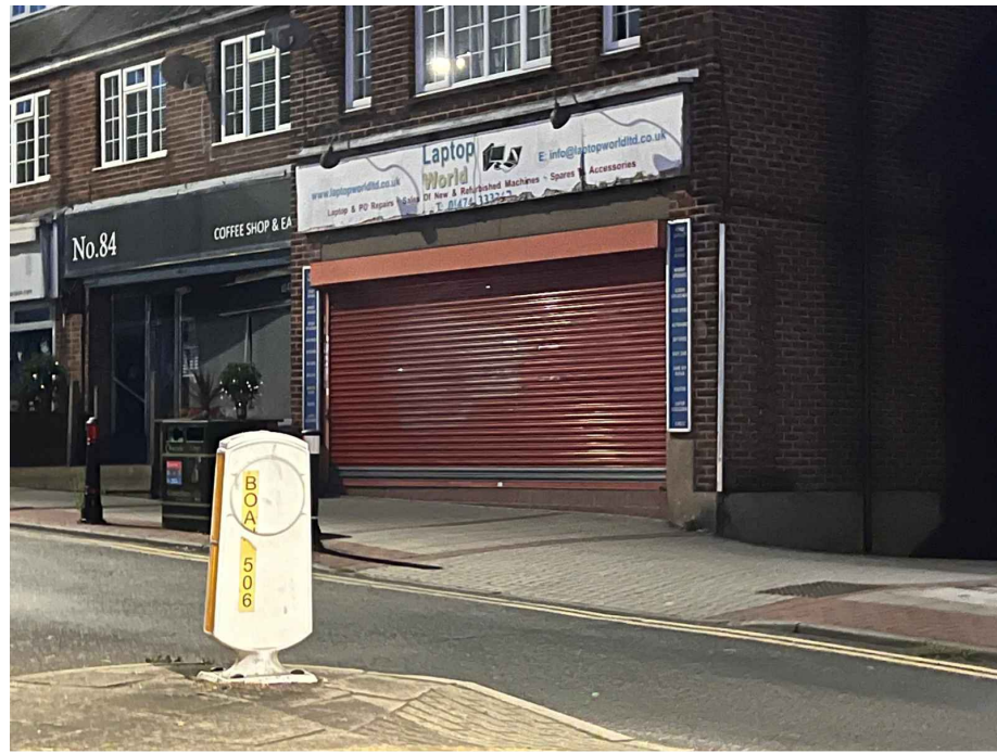
86 Parrock Road Shop Front with Shutter
