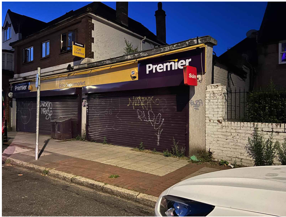
6 Echo Square Shop Front with Shutter
