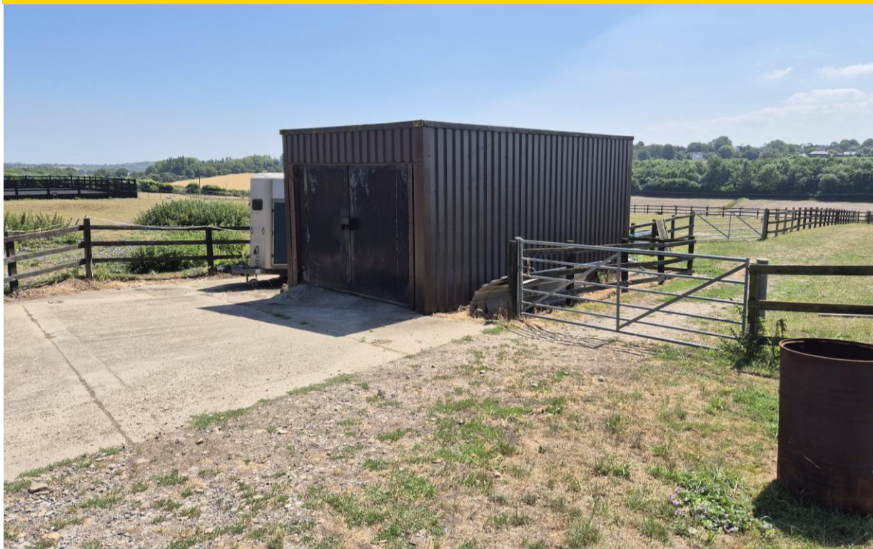
The existing storage container to be relocated.
