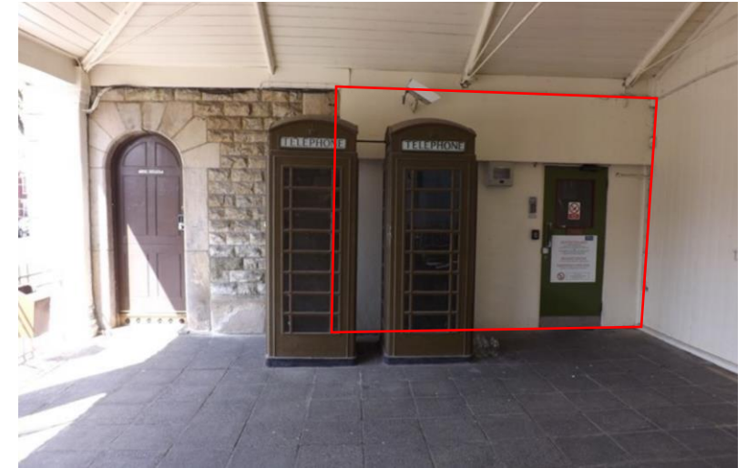
Connection between PCC and Pier – Pier undercroft
