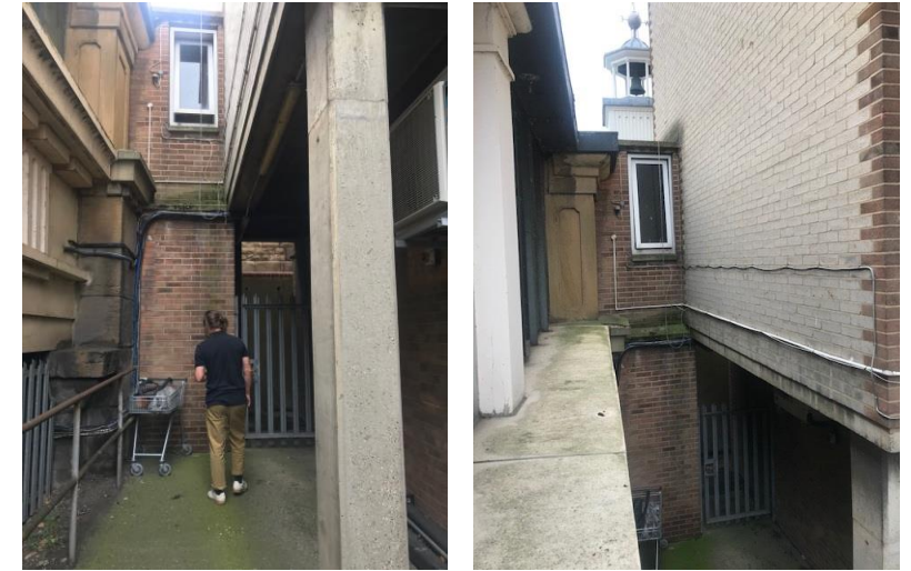
Connection between PCC and Pier – river side
