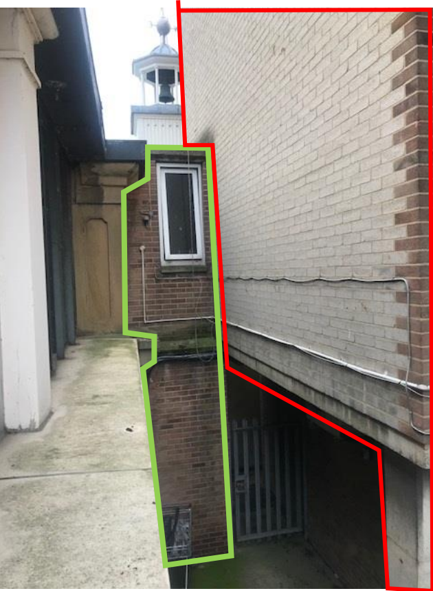
Connection between PCC and Pier – river side
