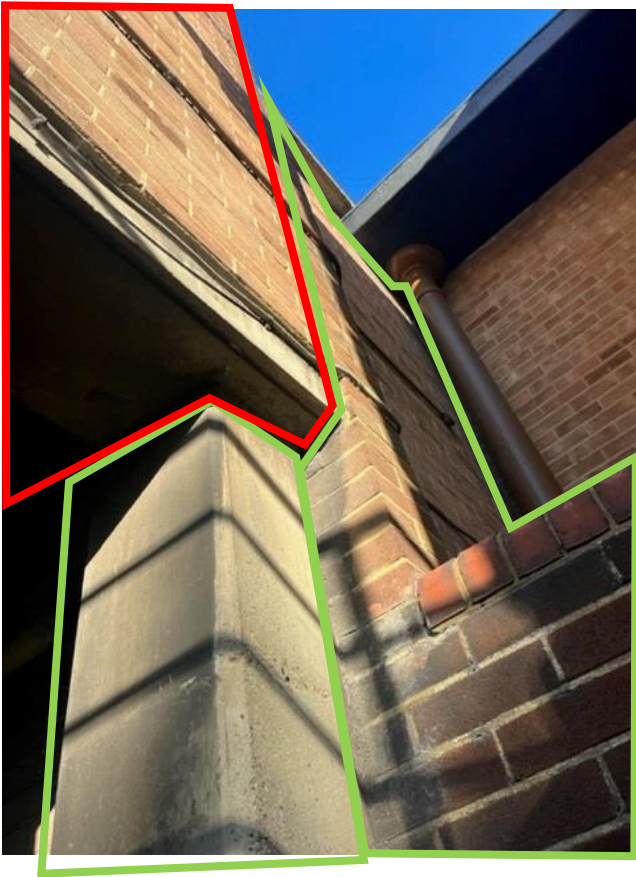
Connection between PCC and Pier – town side, hidden behind Pier
