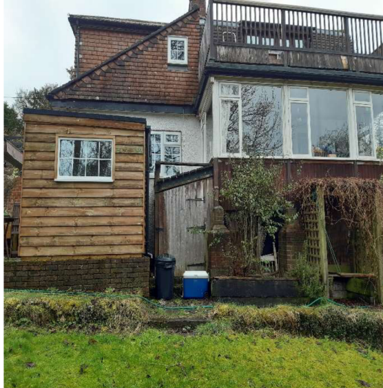
Photo 2 rear of property
