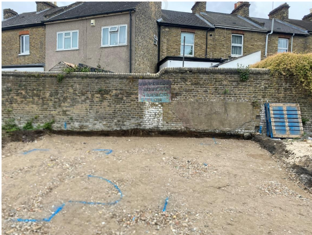
PLAQUE LOCATION AS SEEN APPROACHING FROM ARMOURY DRIVE
