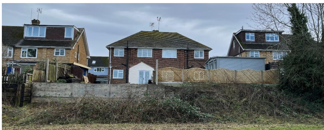
Rear of No.40
