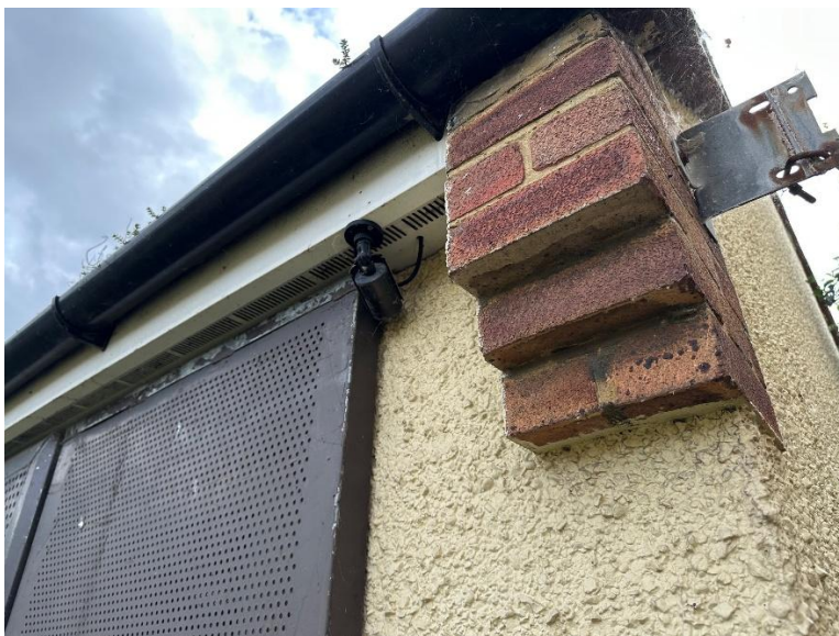
FIGURE 3 – SOFFIT & CORNER OF THE BUILDING
