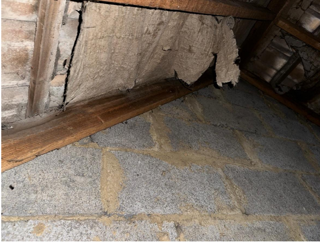
FIGURE 6 – CONCRETE BLOCKS WITHIN THE ATTIC ILLUSTRATING ABSENCE OF BAT ACTIVITY
