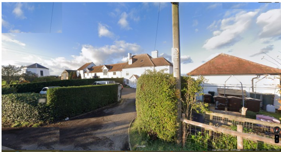
Fig .8. View of front of site from road edge
