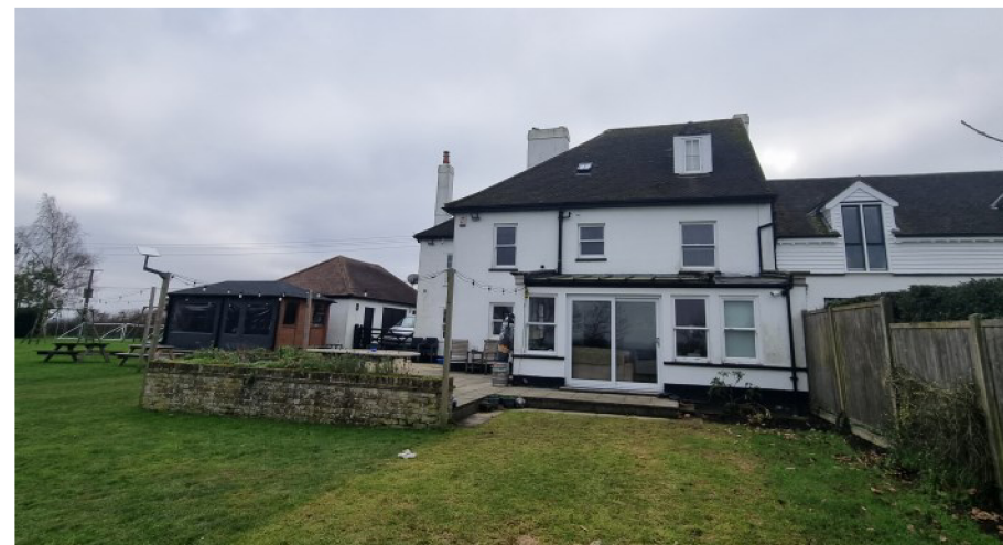
Fig .9. Rear view of Mill House
