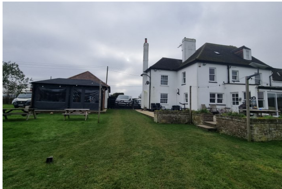
Fig .7. Rear view of Mill House
