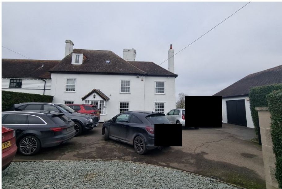
Fig .6. Front view of Mill House
