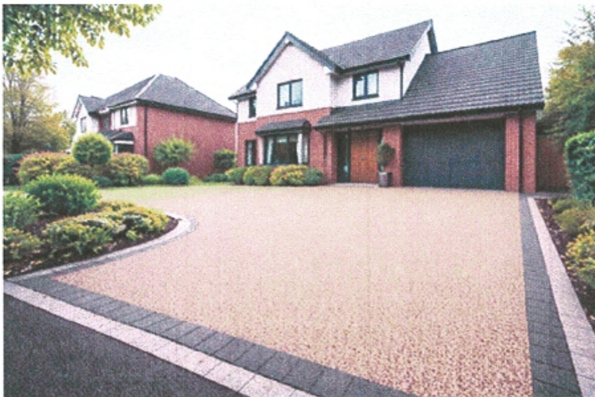
Resin bound gravel drive image
