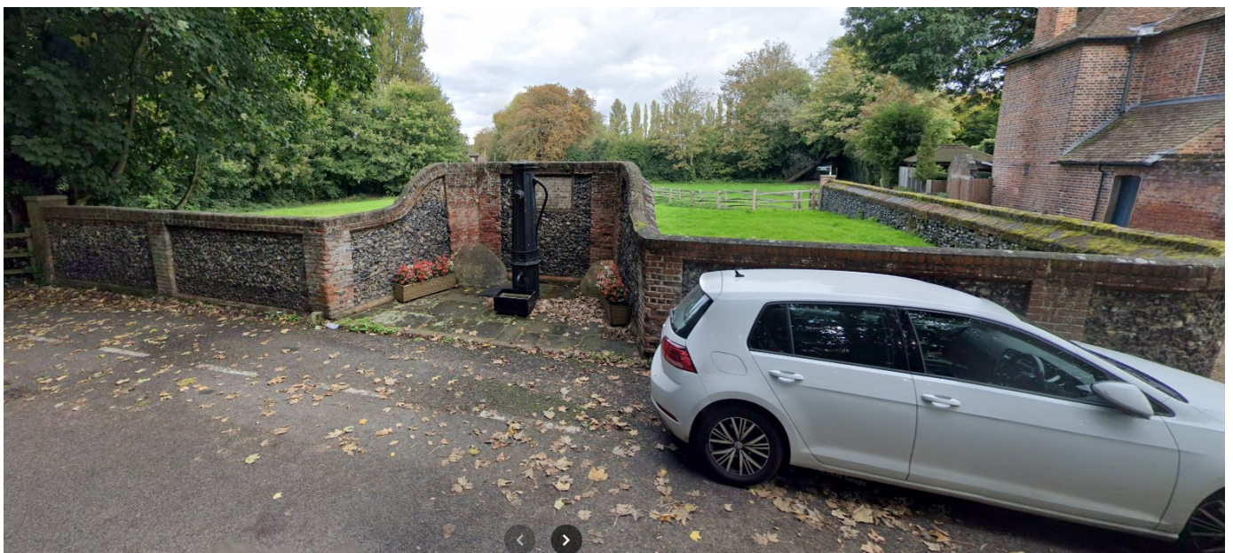
Front of wall
