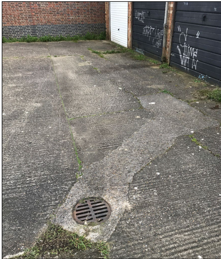
Figure 4.1 – Existing gully on site discharging surface water runoff from the garages and the area of hardstanding.
