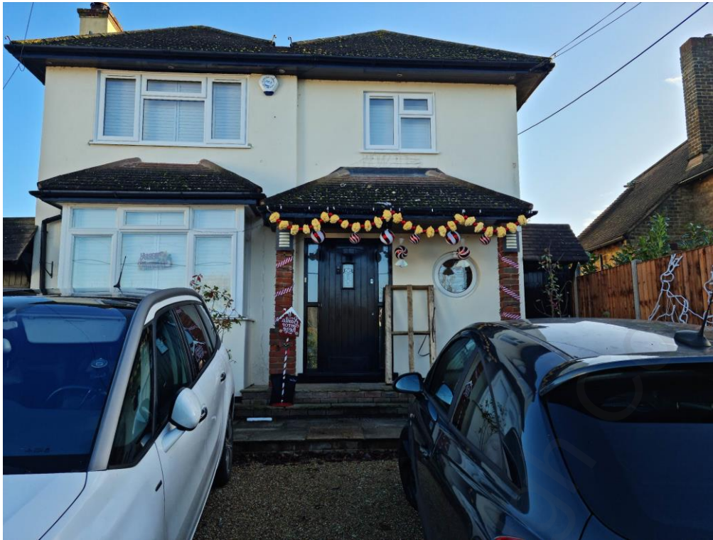
Photo 5 – View of the front of the main dwelling
