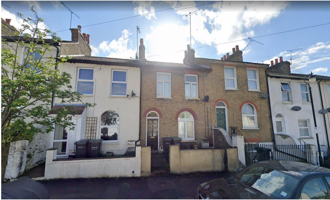
Fig 2: Variety of staggered building heights along Peacock Street, and a mix of yellow stock bricks and rendered facades.
