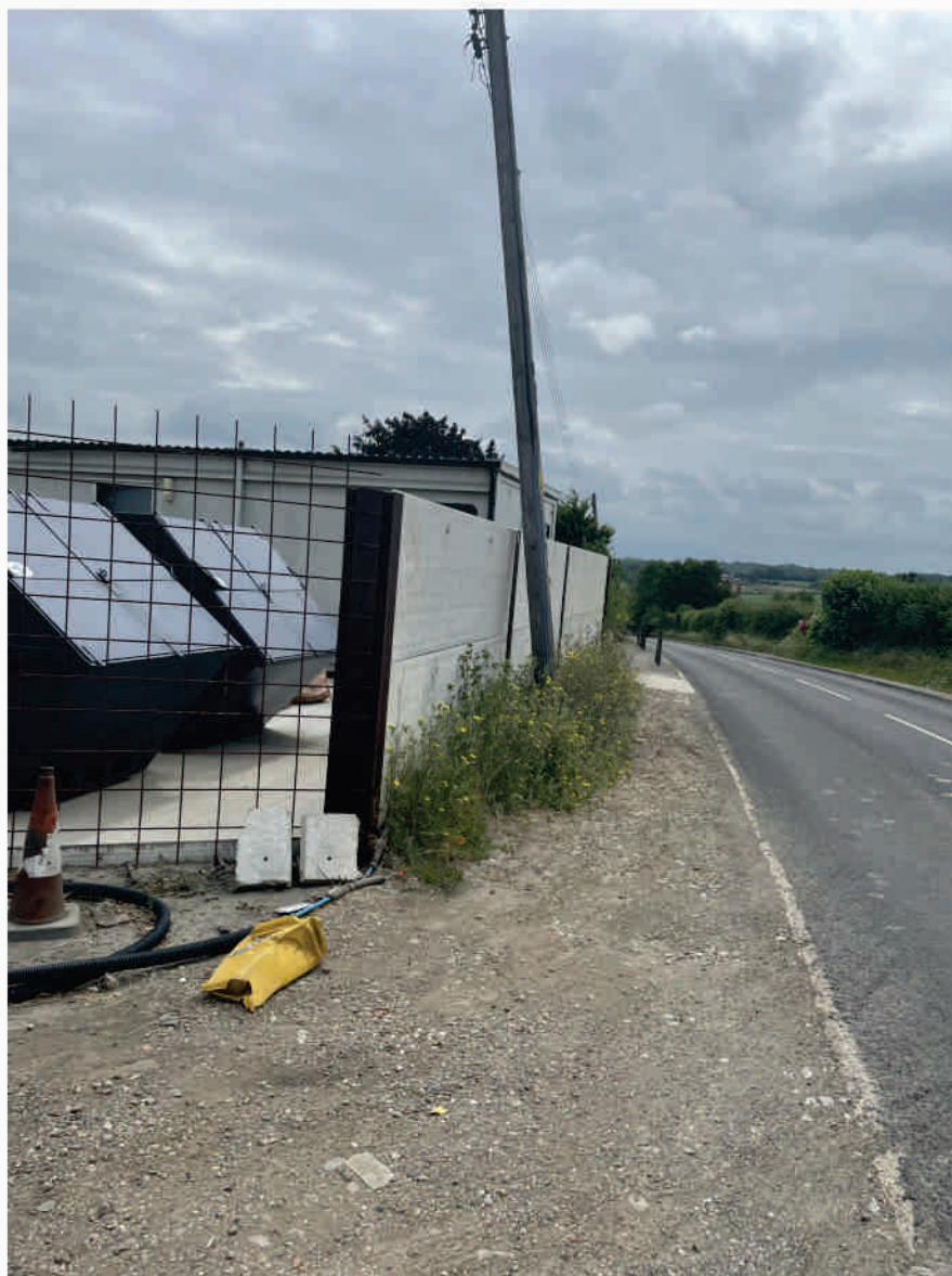
PHOTOGRAPH OF INSTALLED FENCE FROM YARD ENTRANCE
