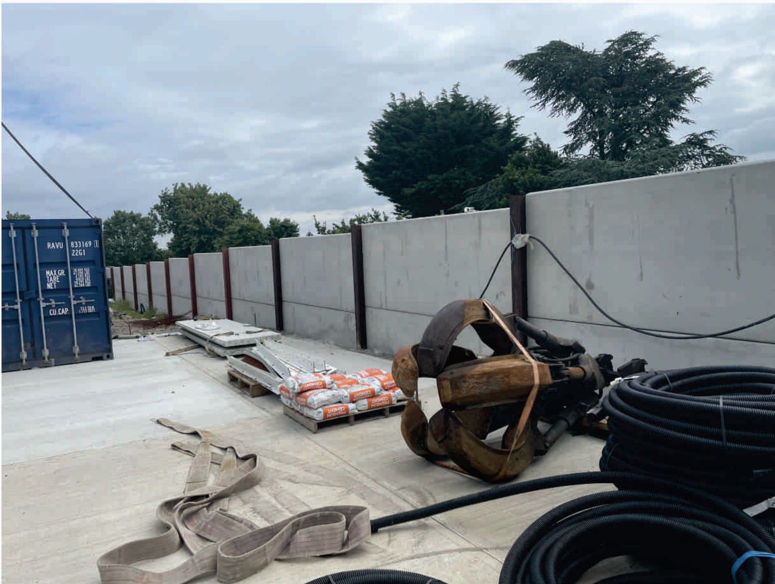
PHOTOGRAPH OF INSTALLED FENCE FROM YARD AREA
