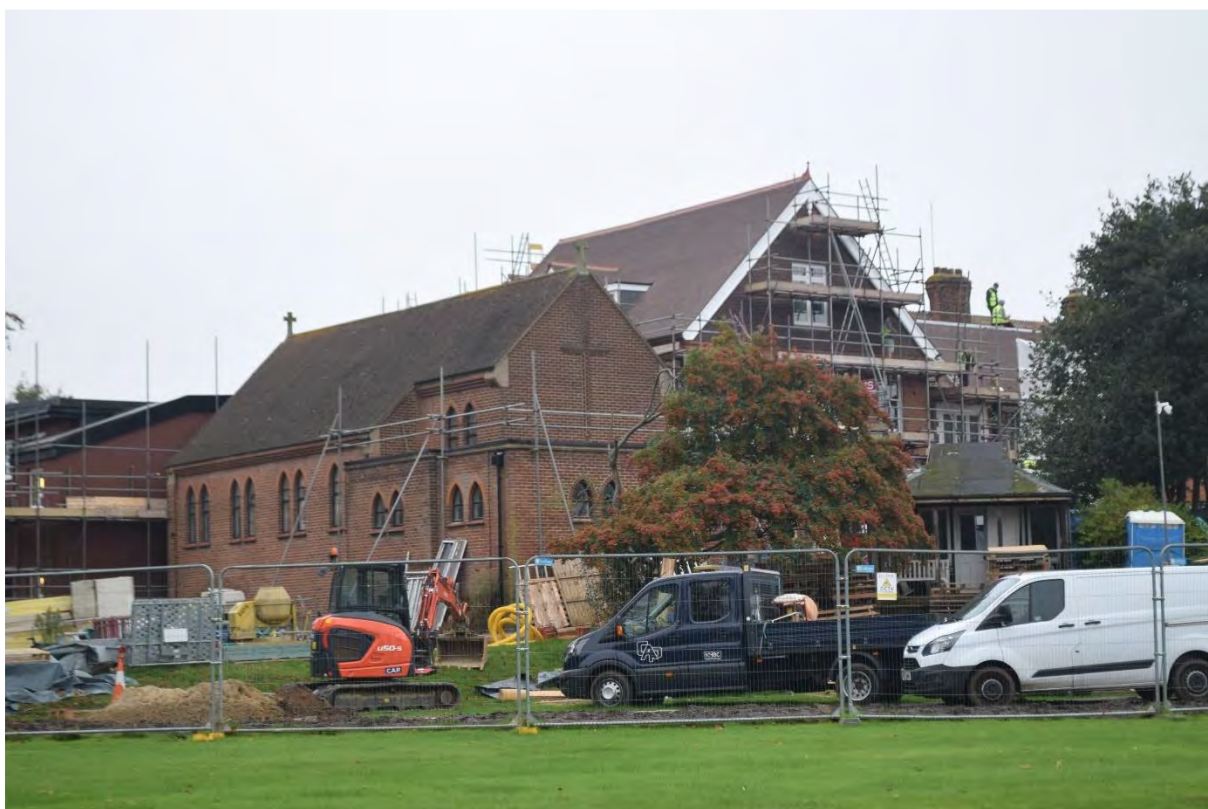
Figure 22. View showing the twentieth century church structure, looking south-west
