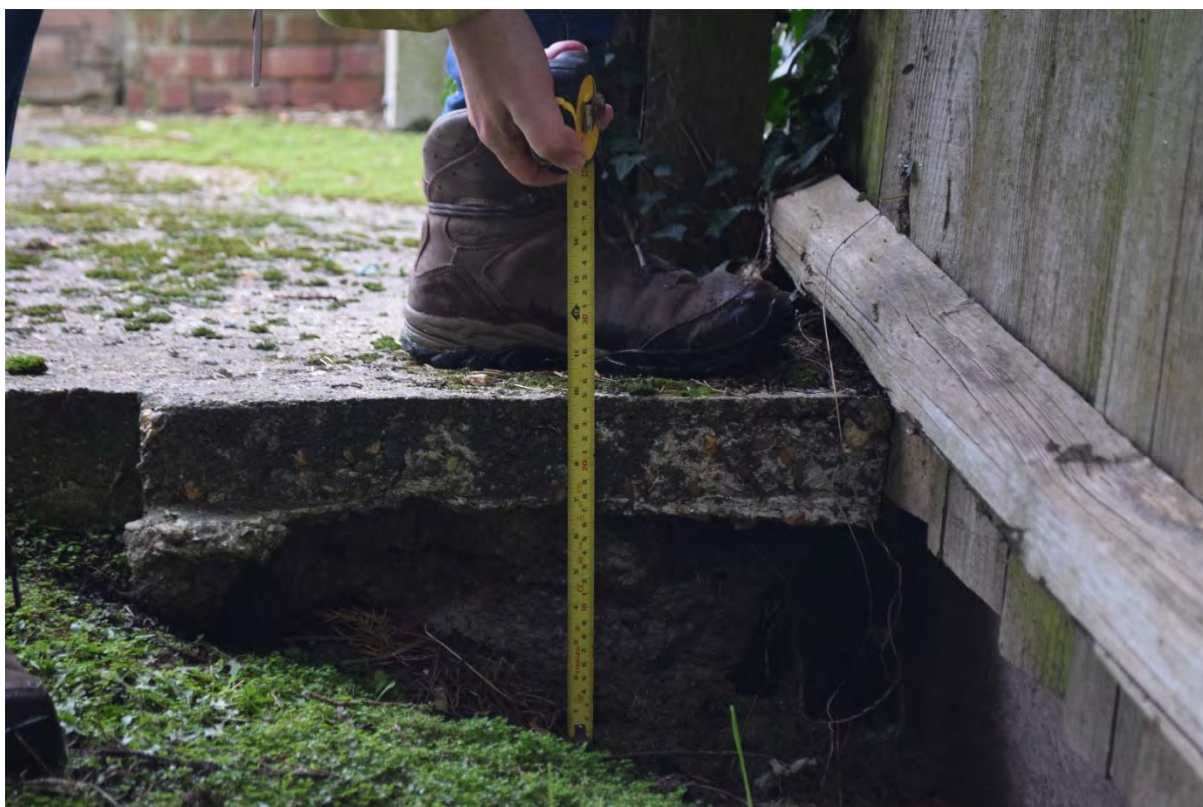
Figure 37. View of the depth of concrete foundations underneath greenhouses, looking south-west
