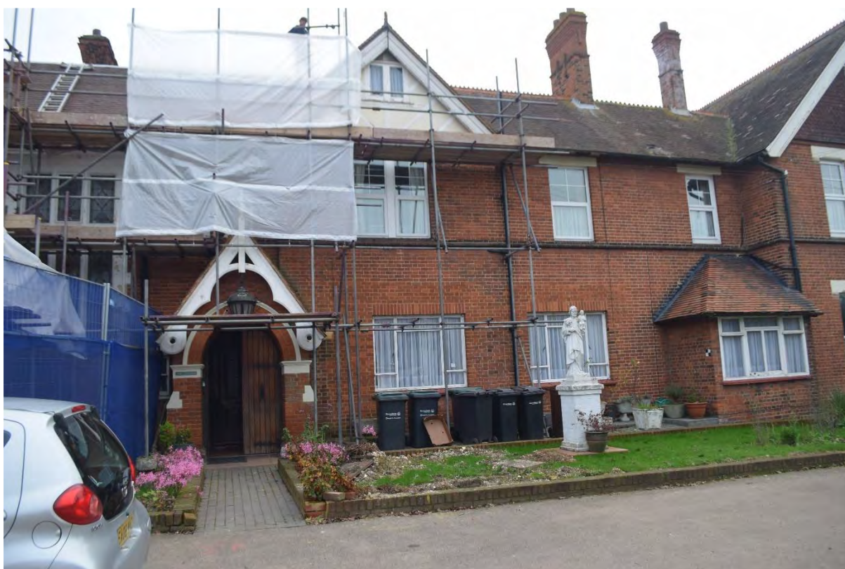
Figure 18. View showing the nineteenth century building, looking south
