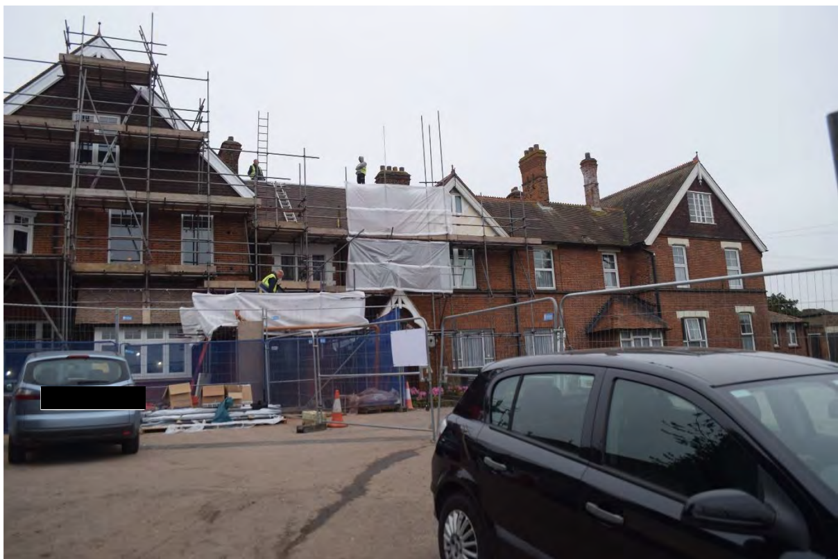
Figure 16. View showing the nineteenth century building, looking south
