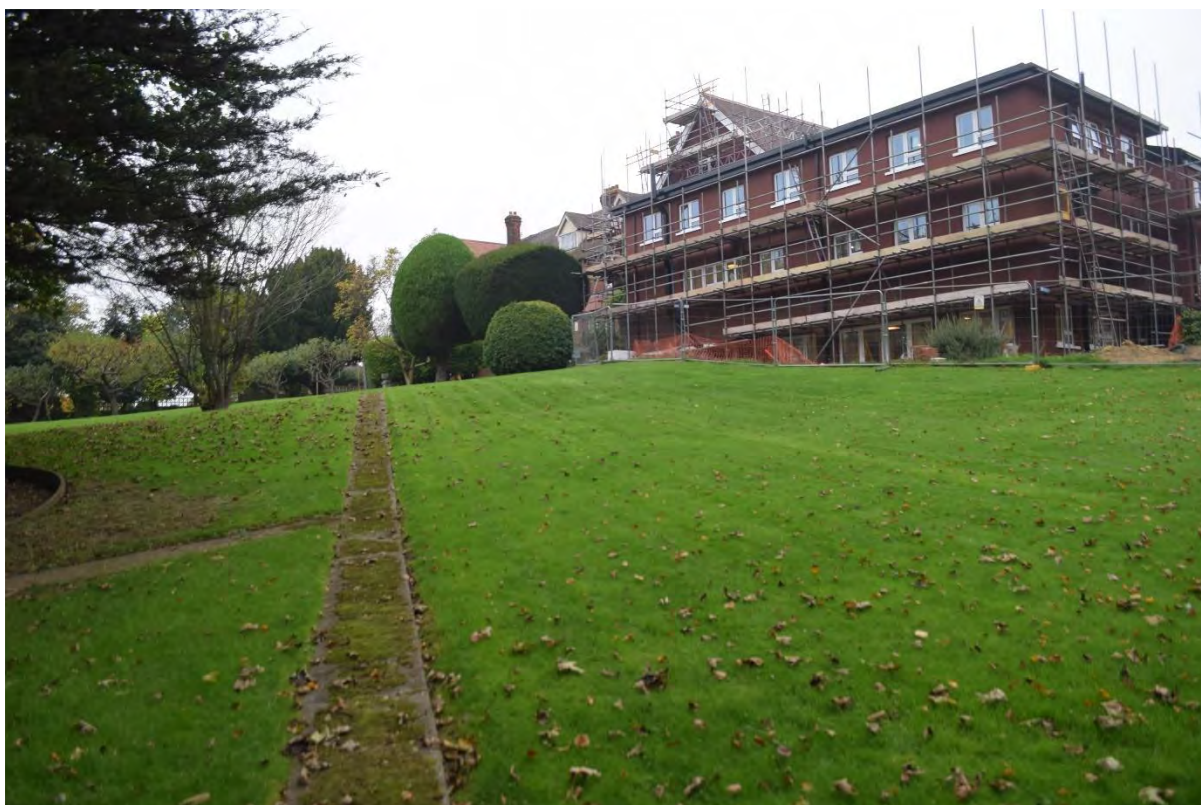
Figure 23. View showing the modern extension, looking north
