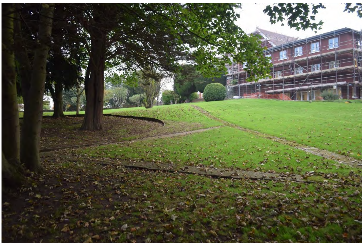
Figure 5. View showing the changing in levels, looking north.
