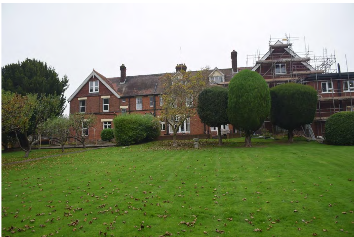
Figure 17. View showing the nineteenth century building, looking north
