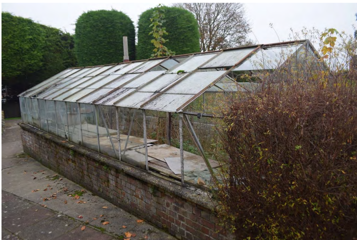
Figure 36. View showing greenhouse with brick foundation
