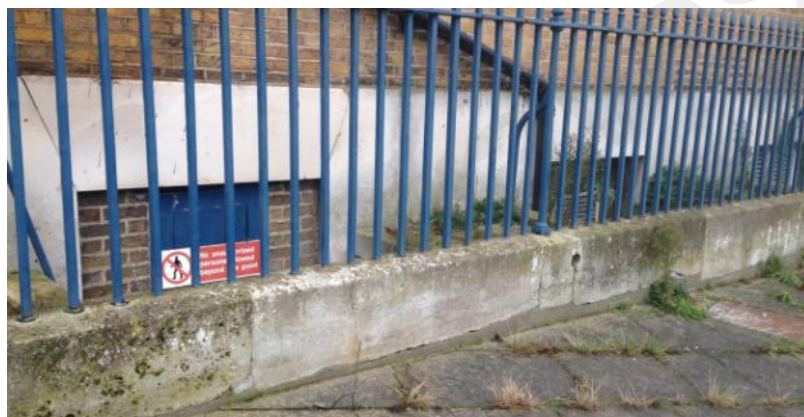
Photo of side elevation light wells
