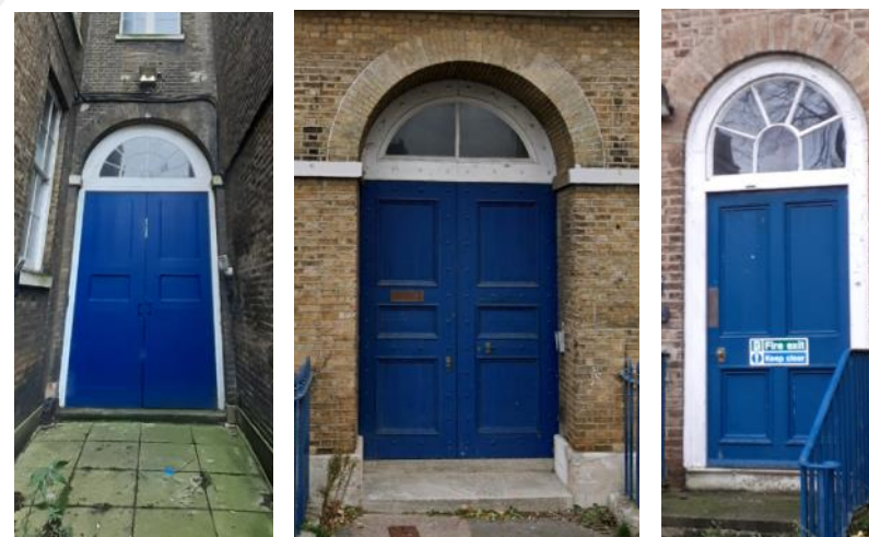
External doors to be refurbished and retained.
