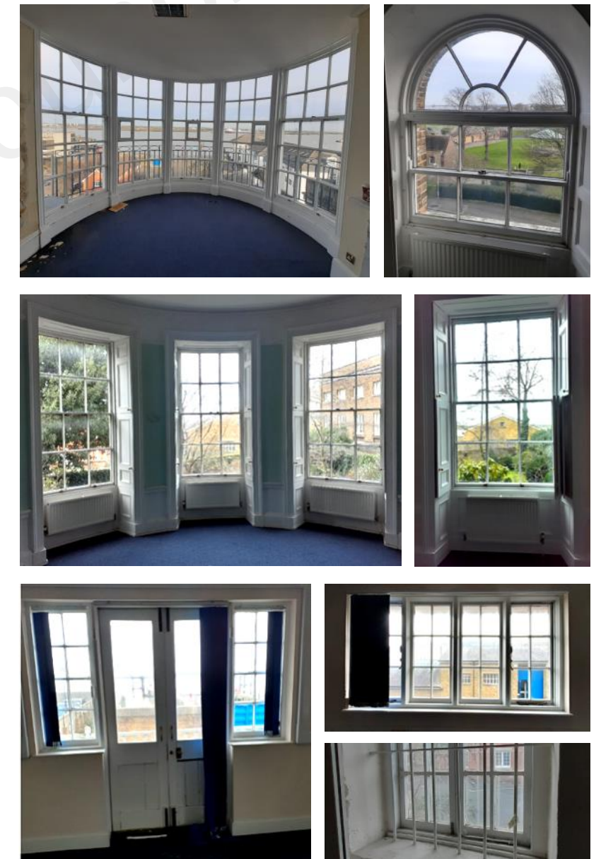
1. Timber, double glazed, large 5-light bow window (lookout); 2. Original single glazed, arched sash window; 3. Original single glazed sash boxes and timber surrounds; 4. Original timber casement sidelights and external door (boathouse); 5. Original, timber single glazed casement window (boathouse); 6. Original, timber casement
