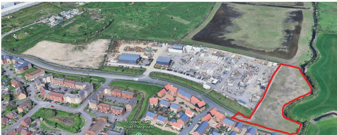
Figure 1 - Aerial Image of site.
