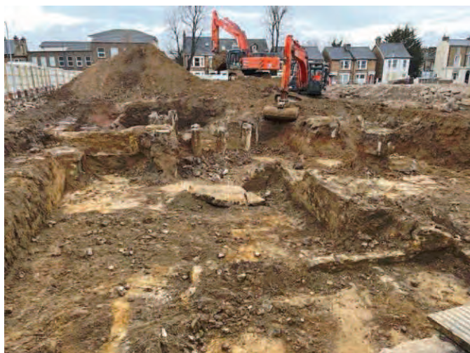
Plate 1: Pile removal west.
