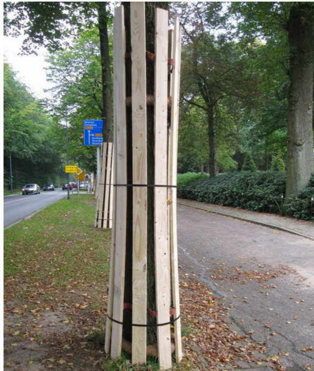
Figure 5 Tree Trunk Protection Measures
