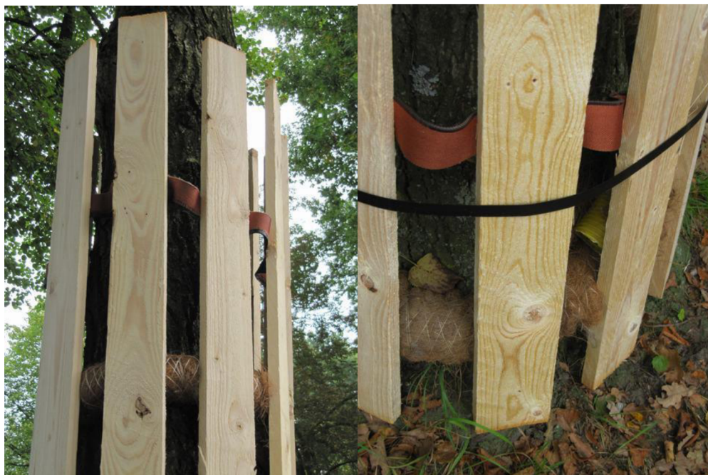
Figure 6 Insulated pipe inside planks, to protect trunk of T01.
