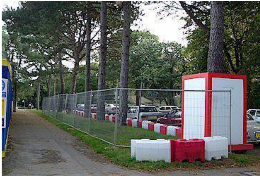
Figure 7 An example of the solid box protection method for tree stems
