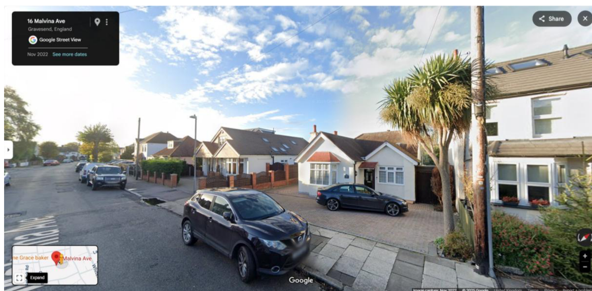
Google Street View of 15 Malvina Avenue and neighbouring properties
