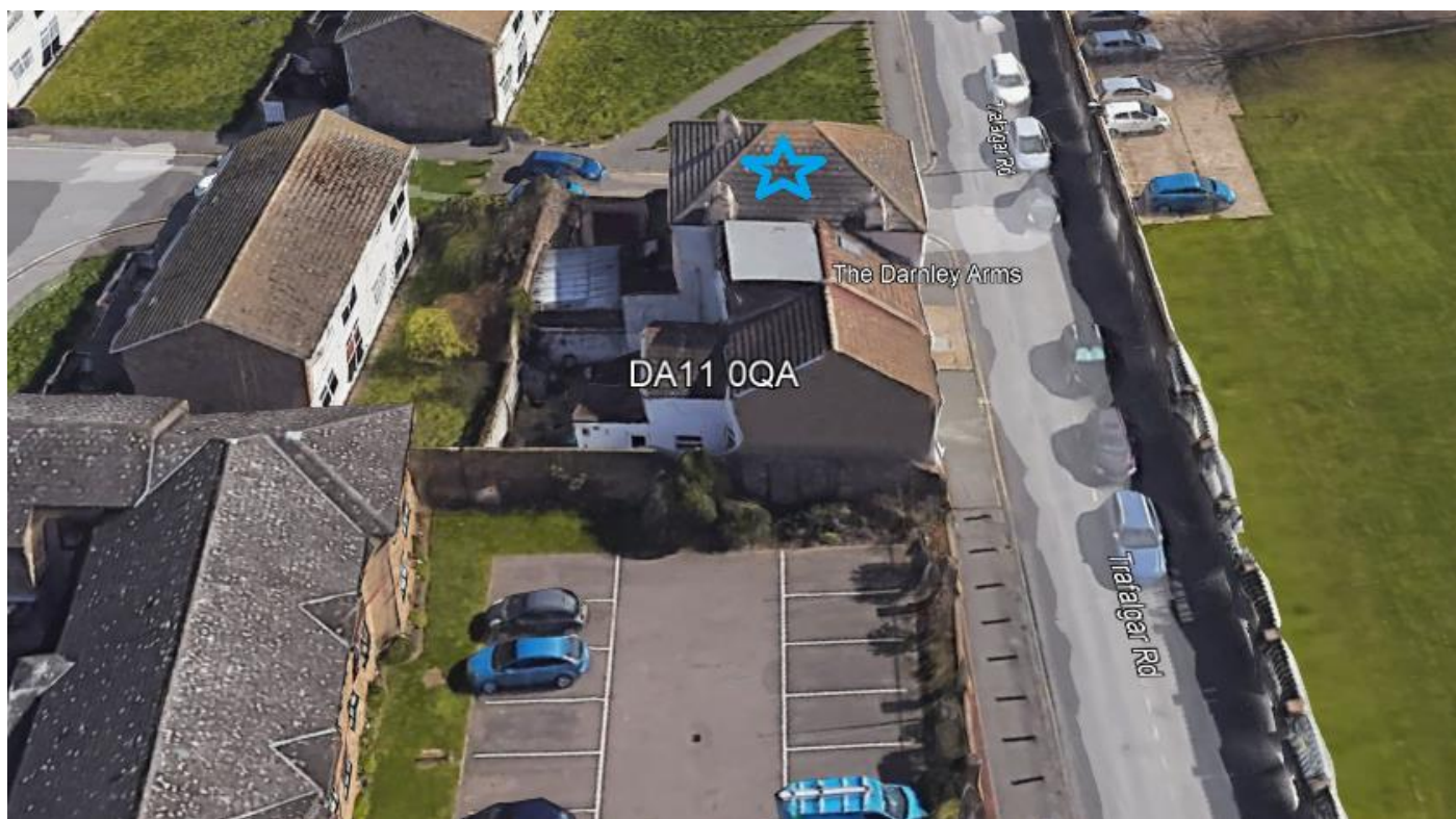
View from the west
