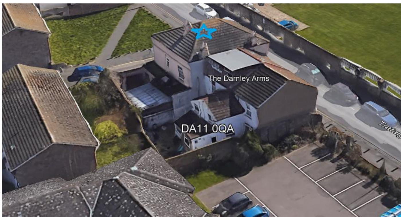
View from the north-west
