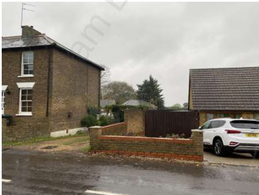
VIEW NORTH-WEST BETWEEN 7 FORGE LANE AND DAVENPEN
