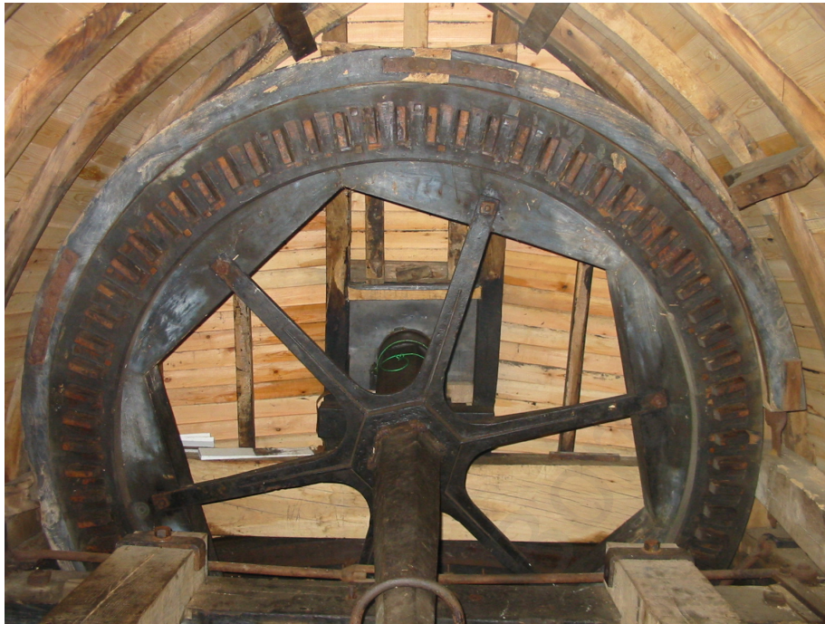
The brake wheel, located inside the cap at the top of the windmill.
