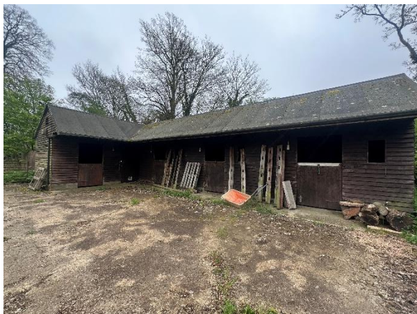
Photograph 4. Stable building on site
