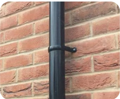
12 Black rainwater goods
