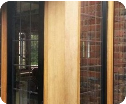
9 Oak Bay window corner details and gablets to projecting gable
