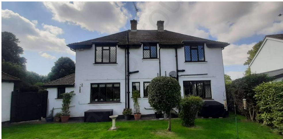
Rear of the house
