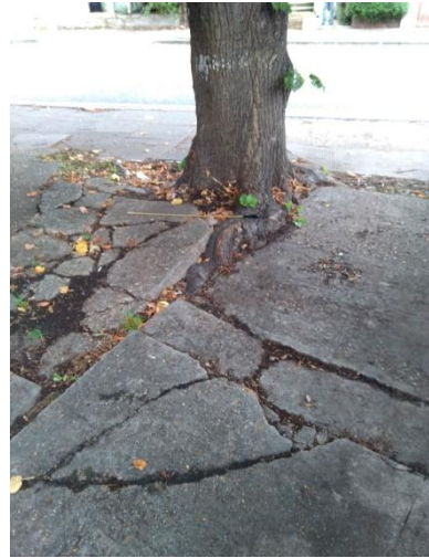
T1 Common lime (Photo 2) - Root damage to the driveway
