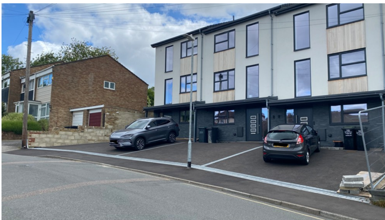
Existing frontage parking arrangements (photograph taken 20 May 2026)
