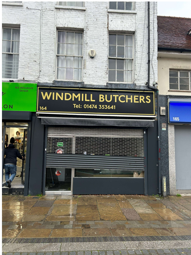
PHOTO – Front entrance to shop to remain as existing.
