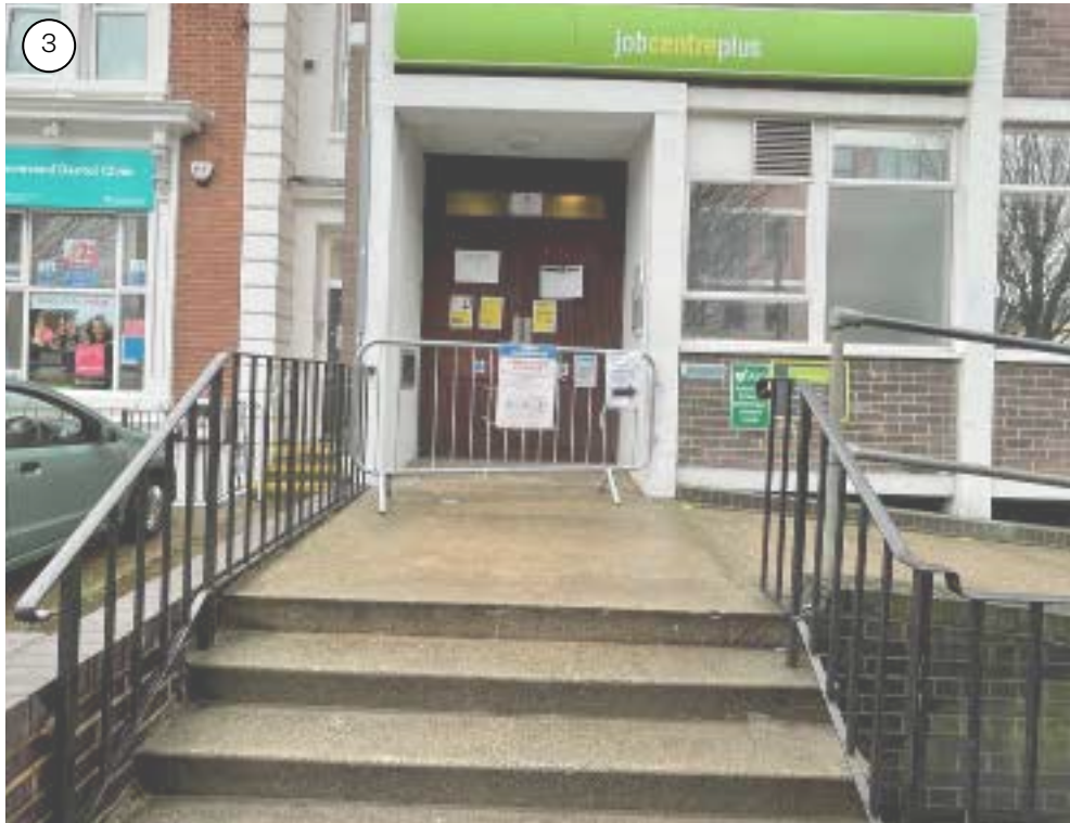
PUBLIC ENTRANCE FROM THE GROVE
