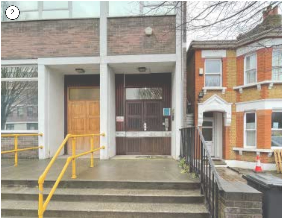
STAFF ENTRANCE FROM THE GROVE
