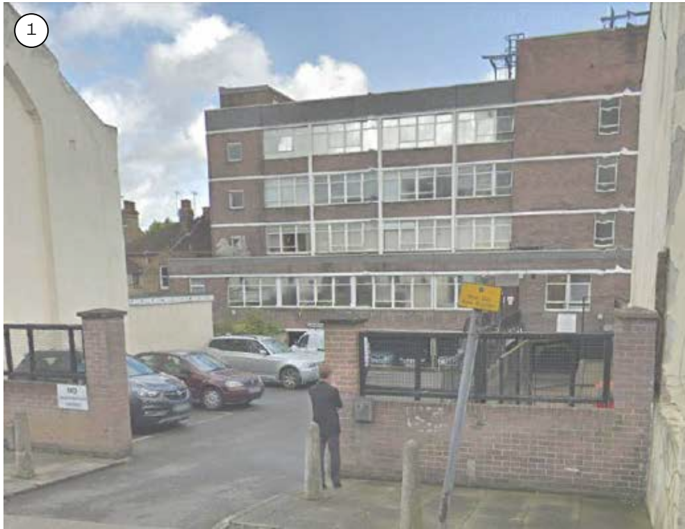
VIEW OF REAR ENTRANCE FROM EDWIN STREET
