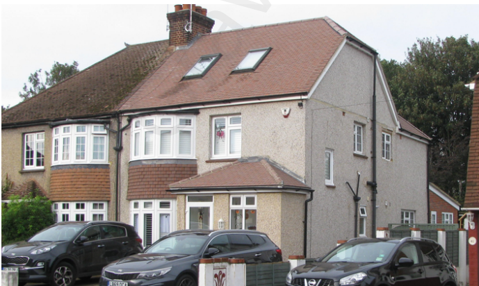
Above: Hip to Gable roof alterations with barn hips at 39 and 17 Milton Hall Road
