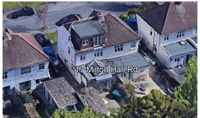
Above: Hip to Gable roof alterations with barn hips at 39 and 17 Milton Hall Road
