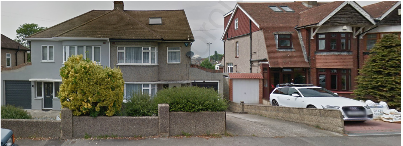
Above: Hip to Gable roof alterations and rear dormers at 55 and 57 Milton Hall Road
