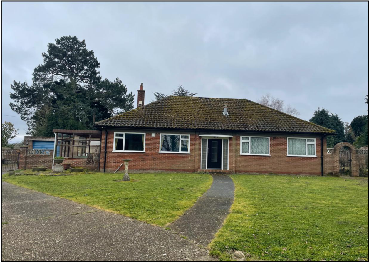
Image taken 16.02.23 – Prior to demolition
