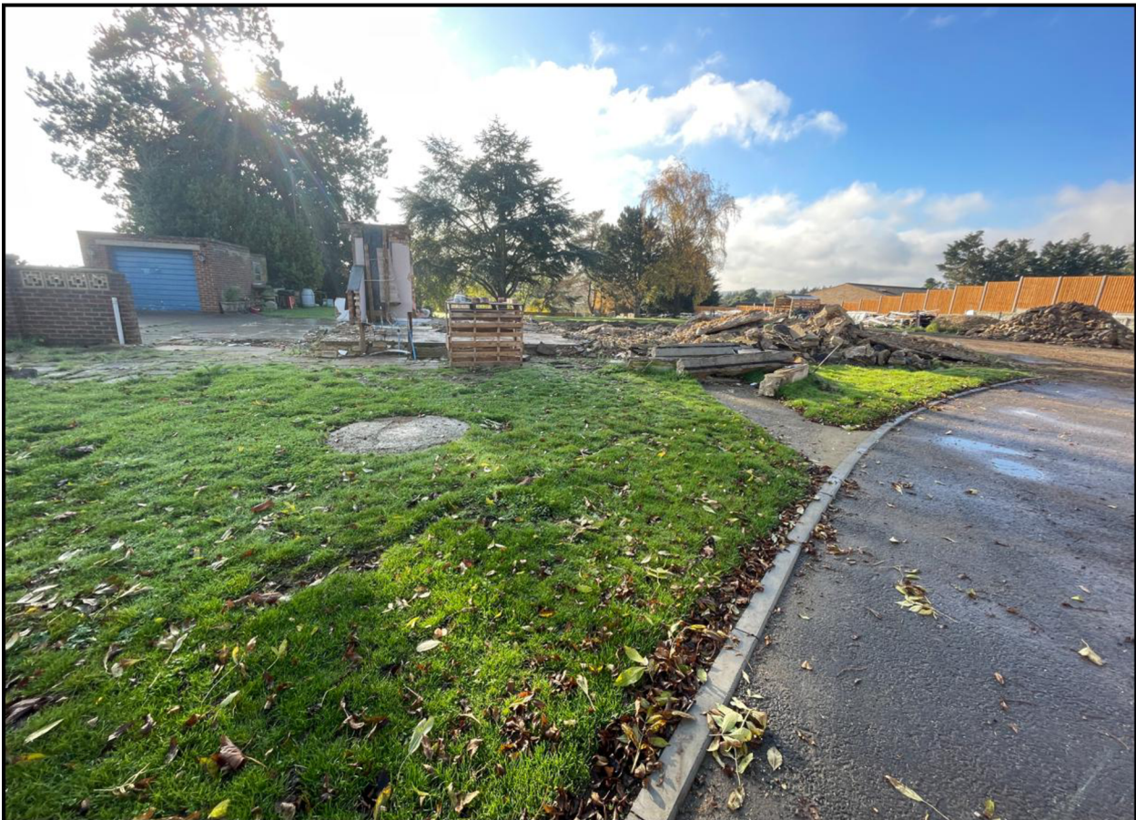
Image taken 14.11.24 – Post demolition
