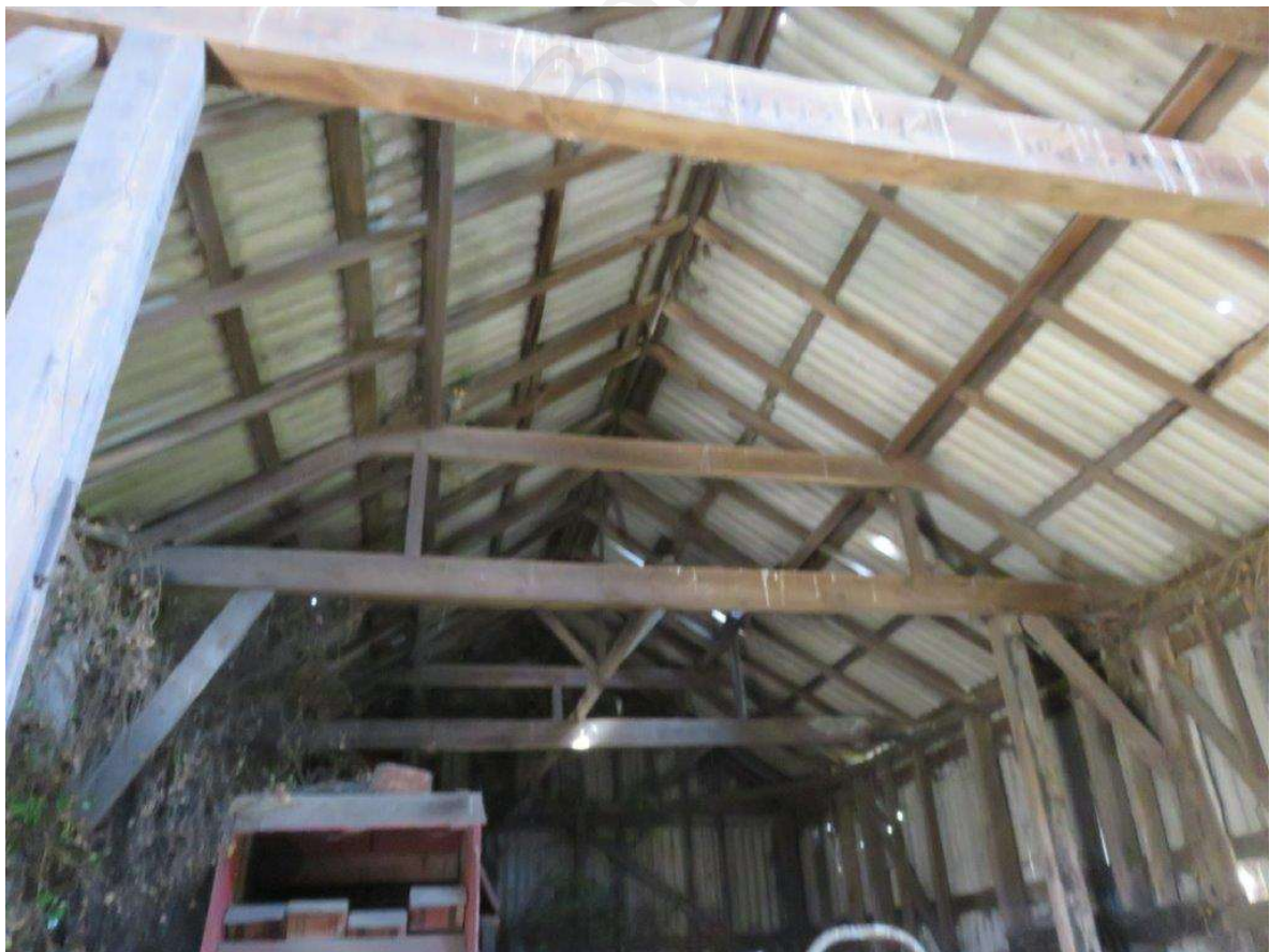
Interior of timber barn
