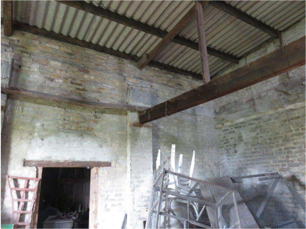
Interior of brick building
