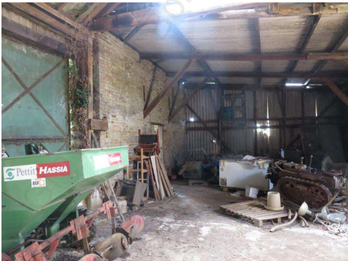
Interior of timber barn – looking towards brick part
