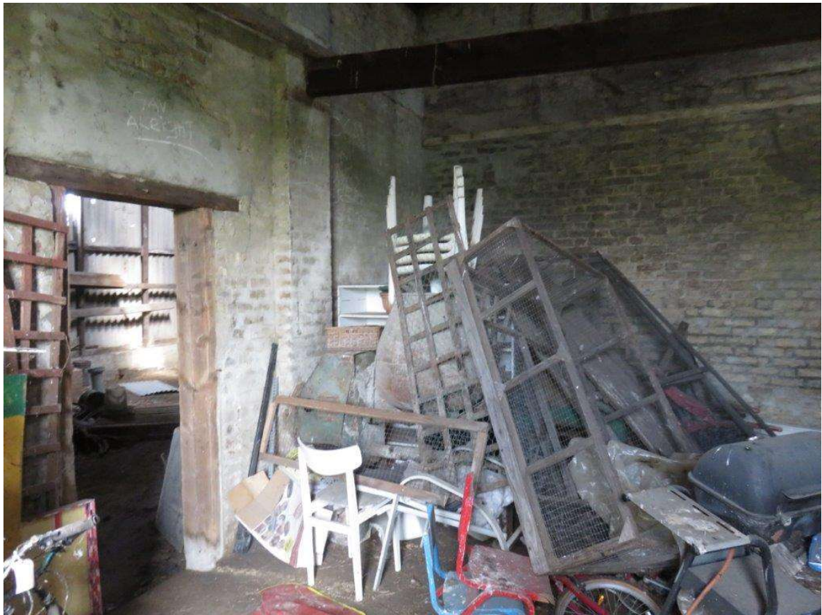
Interior of brick building
