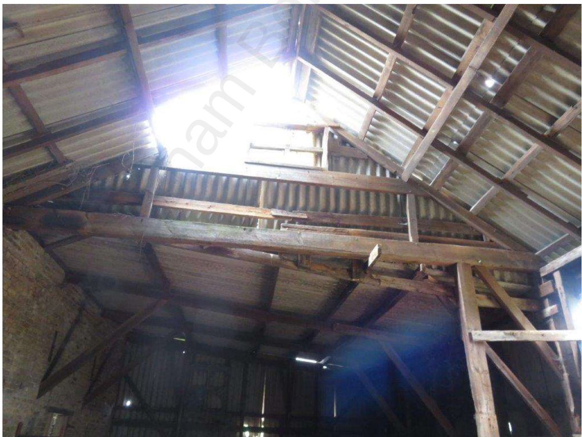
Interior of timber barn junction of pitched and shallow pitched roof
