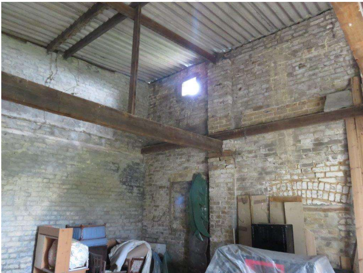
Interior of brick building
