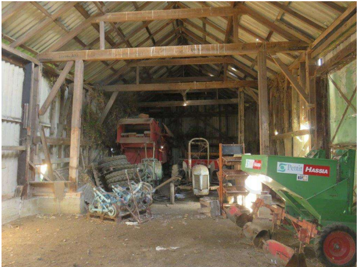
Interior of timber barn
