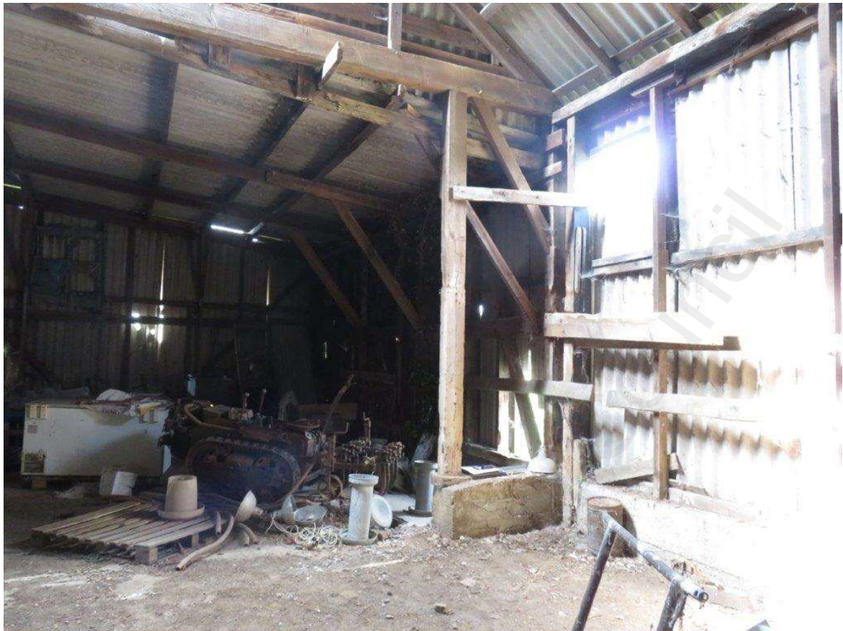
Interior of timber barn
