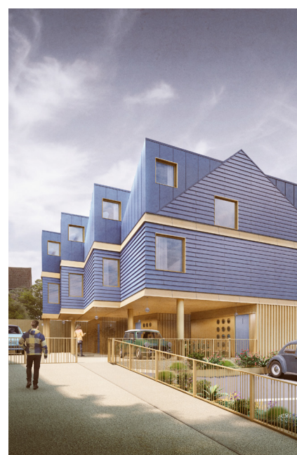
Example of fibre cement planks on proposed facade, using drawings from the Design & Access Statement of the consented planning application. (Right: pg. 48, Left: pg. 44)
