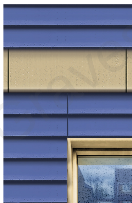
Example of fibre cement planks on proposed facade, using drawings from the Design & Access Statement of the consented planning application. (Right: pg. 48, Left: pg. 44)
